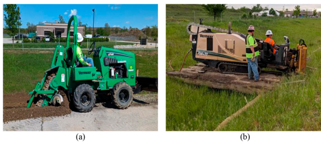
Figure 2.4 Trenching Operations for Conduit Installation: (a) Ride-On Chain Trencher Used for Trench Excavation and (b) Completed Trench Prepared for Conduit Placement.
