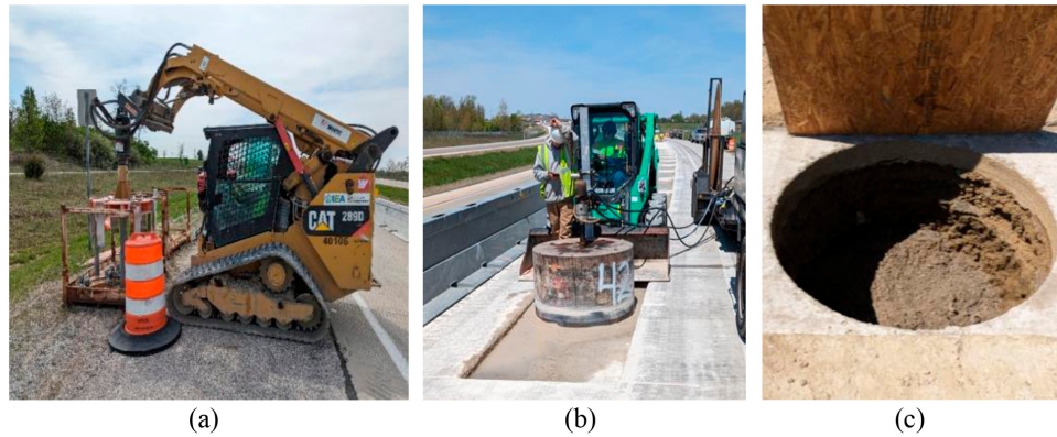
Figure 2.3 Stub-Out Coring Operations: (a) 12-in. Diameter Vertical Core Drilling Using a Hydraulically Driven Coring Attachment, (b) 42-in. Diameter Circular Access Opening Using a Manhole Cutting Head, and (c) Completed Access Opening Within the DWPT Channel.
