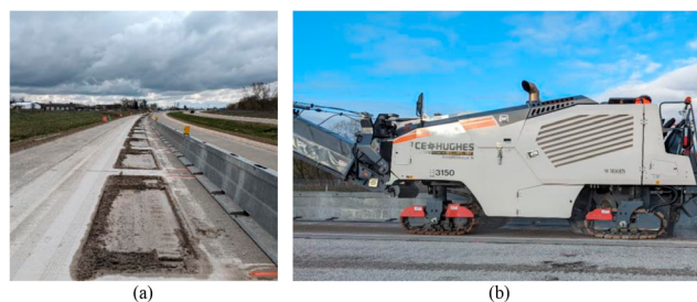
Figure 2.2 (a) DWPT Channel Milling Within PCC Panels and (b) Conventional Milling Machine Used for Channel Construction.
