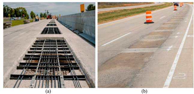
Figure 2.6 DWPT Transmitter Installation and Pavement Restoration: (a) DWPT Transmitter Assemblies Placed Within the Milled Channel Prior to Concrete Placement and (b) DWPT Channel After Polyester Concrete Placement and Surface Restoration.
