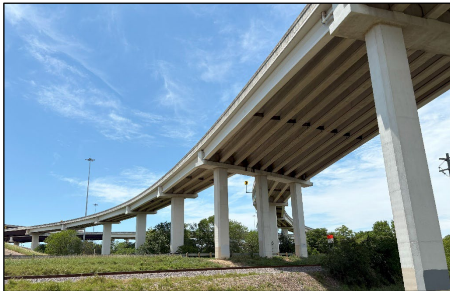
Figure 2.4. Complex multi-level interchange in Austin, Texas, with large portions using simple span and continuous deck construction
