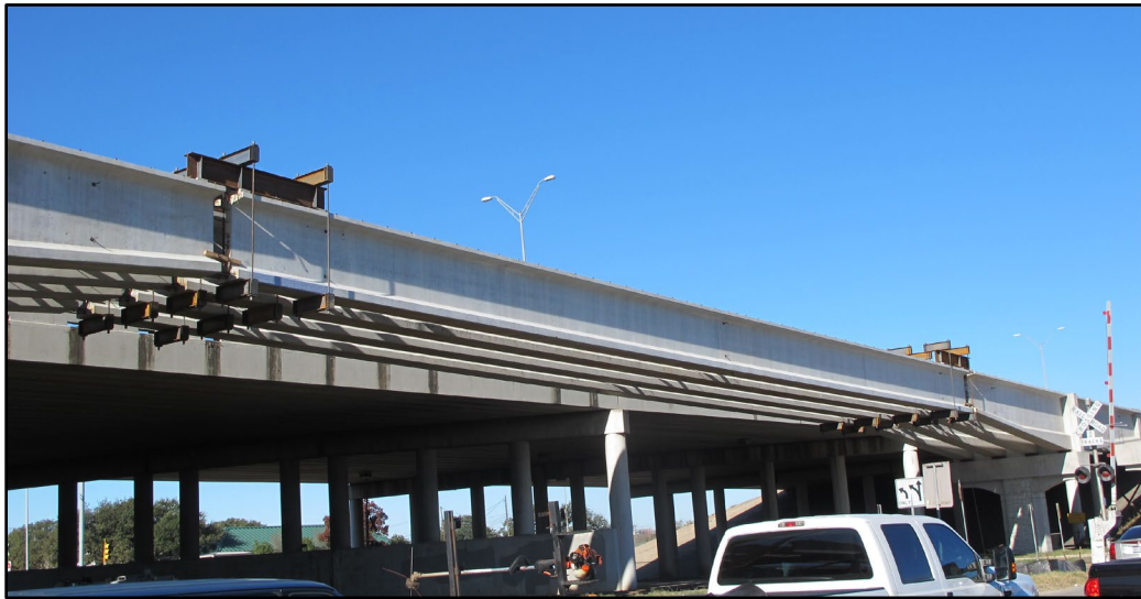
(a) Main span of bridge under construction, Ge et al. (2019)
