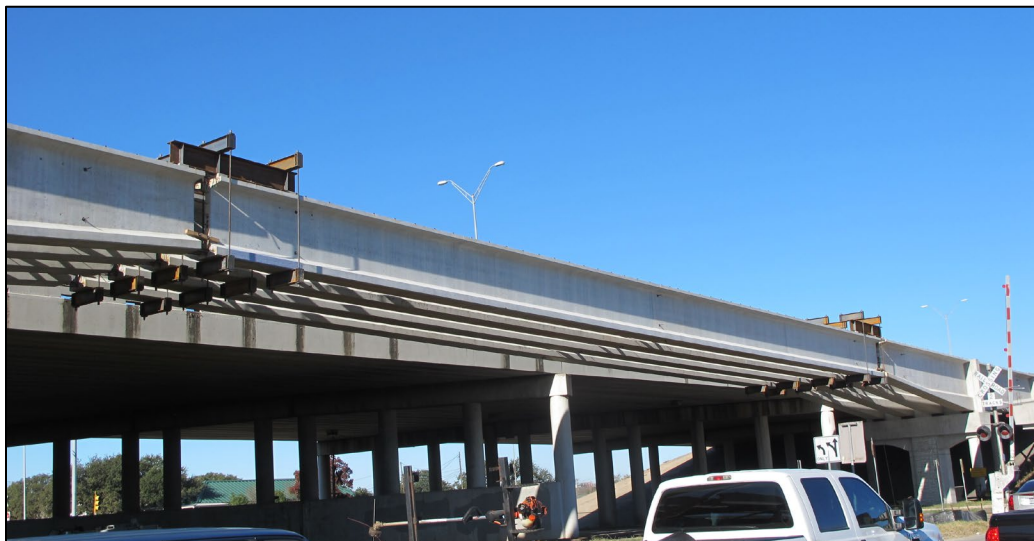
(a) Elevation of main span during construction, Ge et al. (2019)
