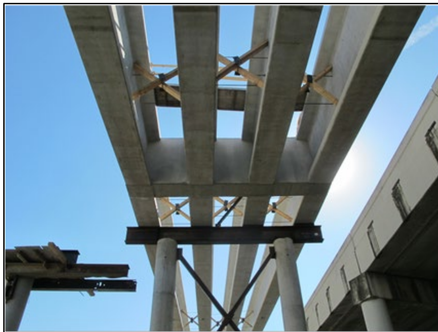
Figure 1.2. Cast-in-place diaphragms at splice locations
