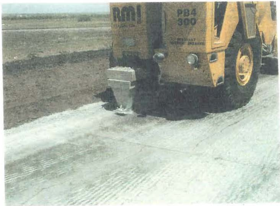
Figure 5. Resonant Breaker
