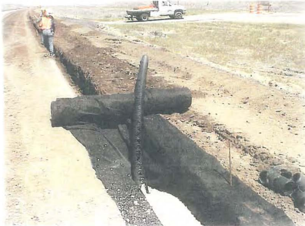
Figure 3. Typical Edge Drain Construction
