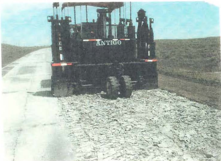
Figure 6. Multi-head Hammer
