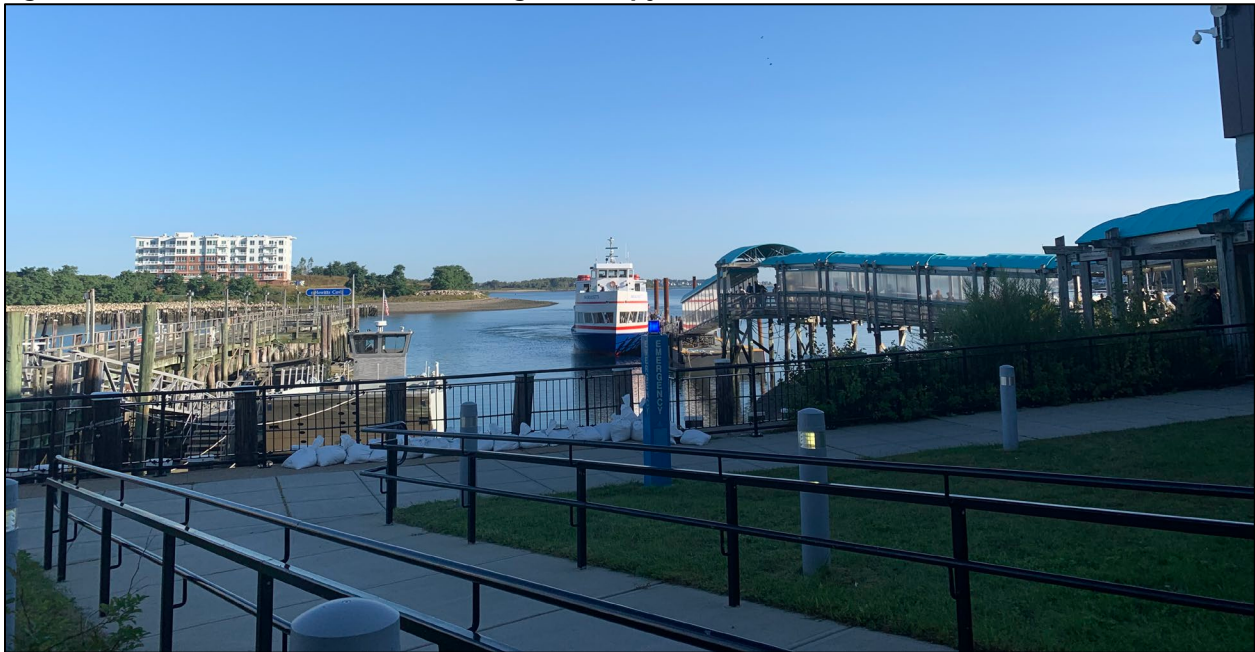
Figure 14: Port dock infrastructure at Hingham Shipyard.
