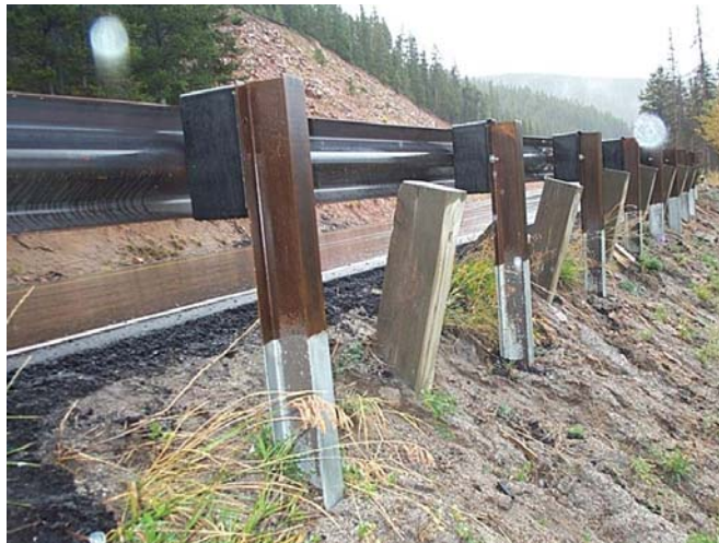
Figure 4. US-50 has steep slopes to both sides.
