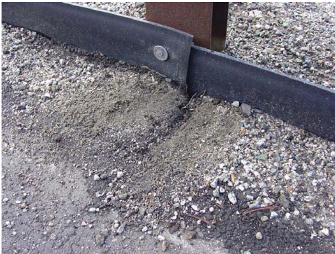
Figure 17. DFC nailed to a guardrail post on US-50.
