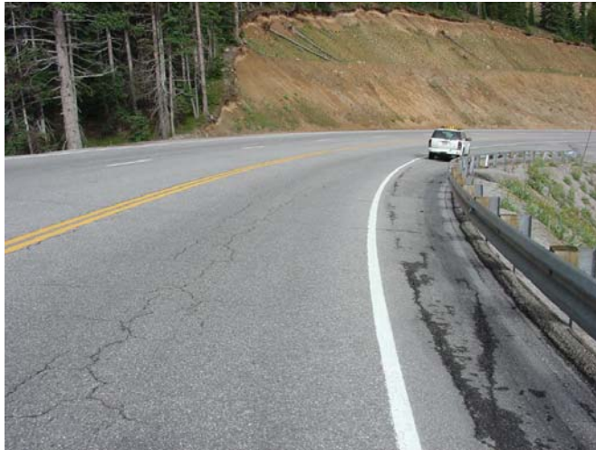
Figure 22. Wide highway and steep shoulders.
