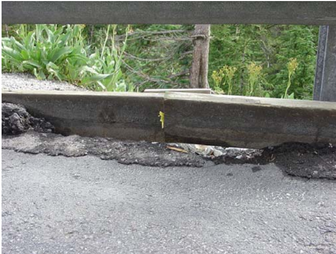
Figure 3. Wood curb can twist and warp.
