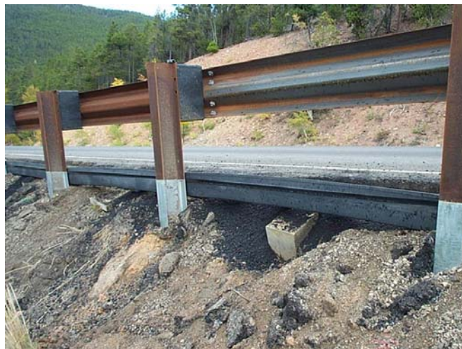
Figure 23. Slopes start under the guardrail.
