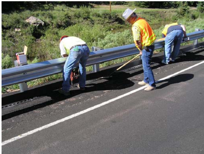
Figure 10. Holding DFC tight against the post base and the pavement with a shovel.
