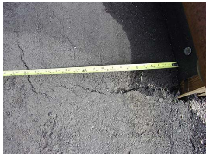
Figure 15. Cracks are developing at the end and along the edge of the DFC on US-50.
