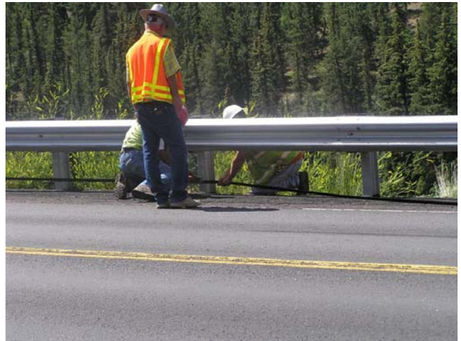
Figure 13. Steel band was installed to provide support for the DFC between posts.
