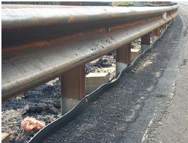
Figure 6. The edge of the pavement was placed and compacted by hand.
