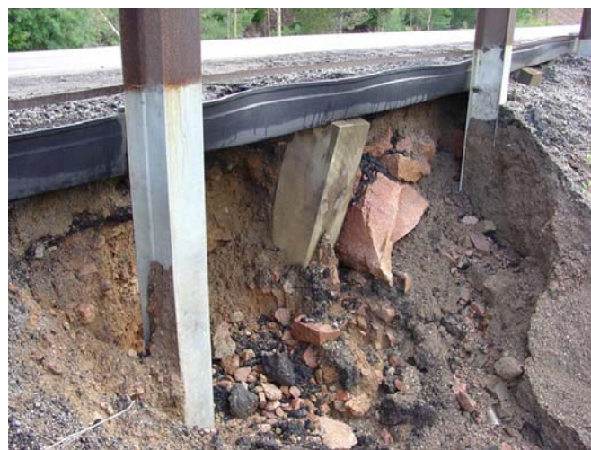
Figure 9. Without the support of the DFC, the edge of the pavement would have collapsed.
