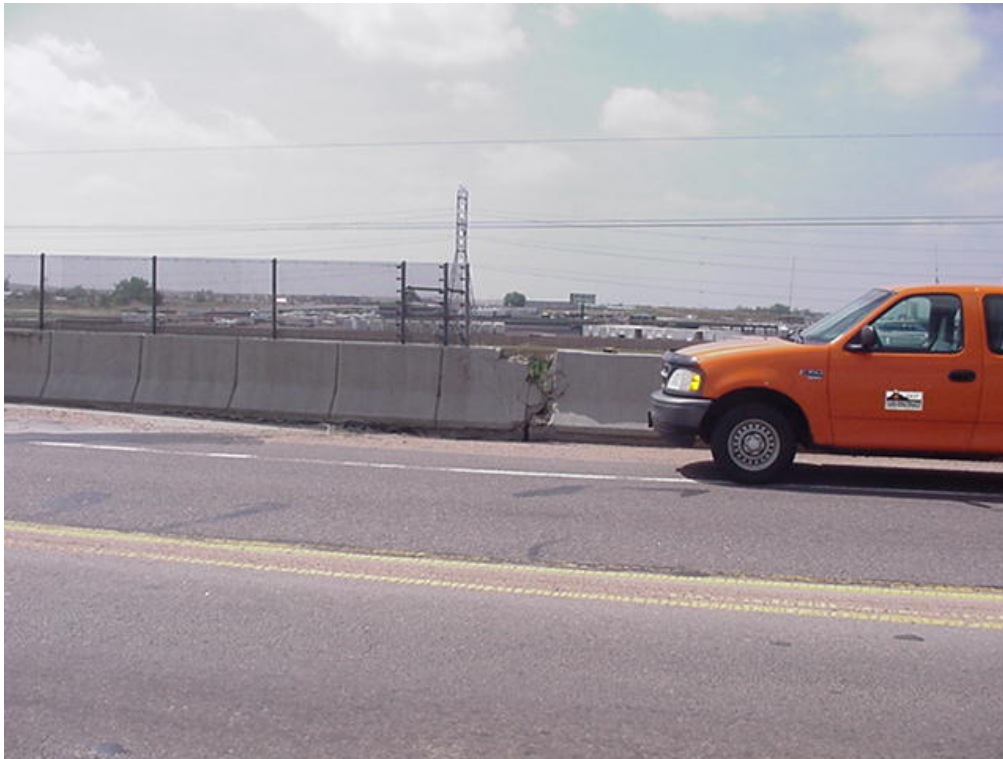
Figure C.10. Photos of Structure E-17-VR in Region 6
