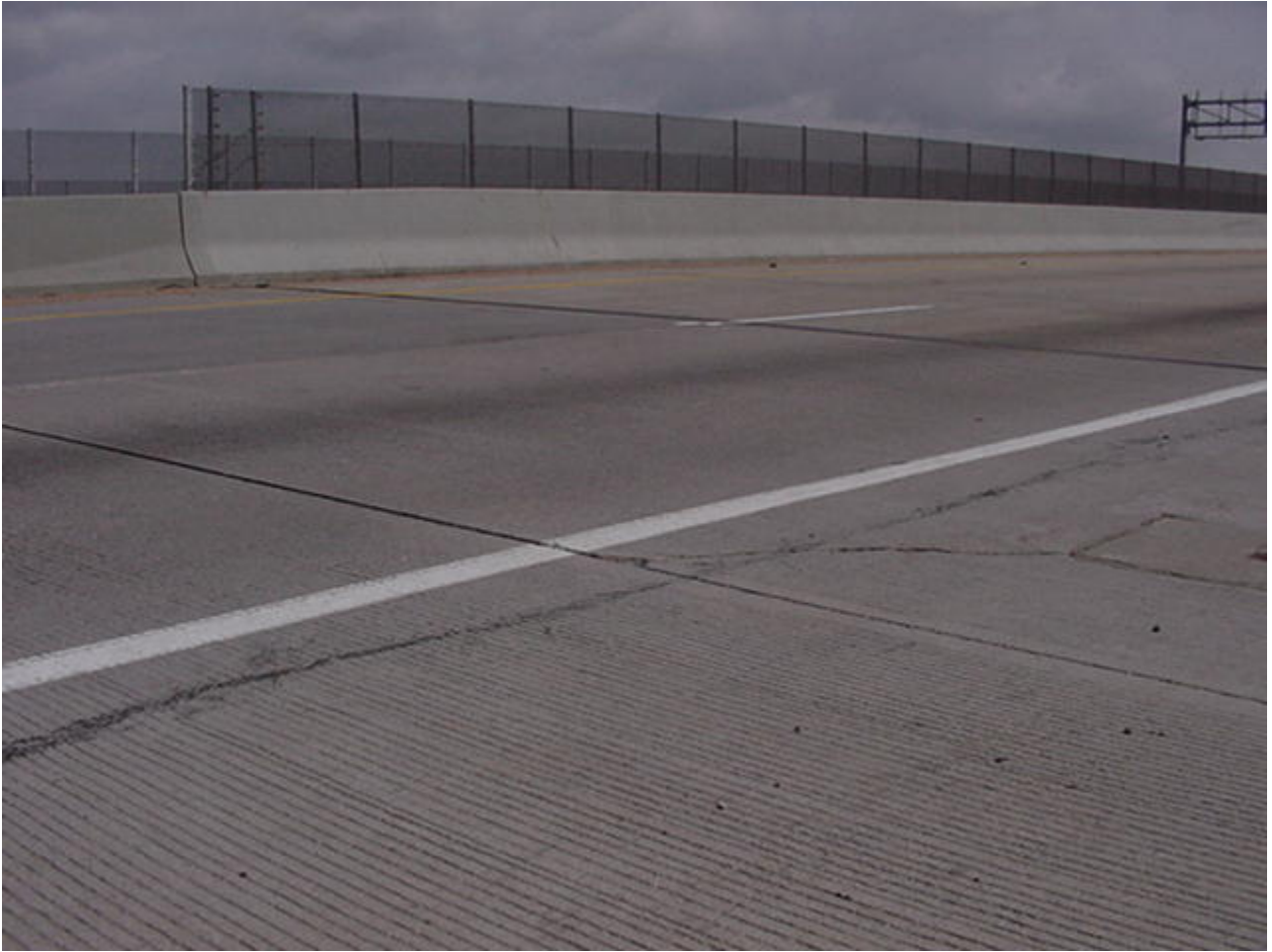
Figure C.9. Photo of Structure E-17-PS in Region 6
