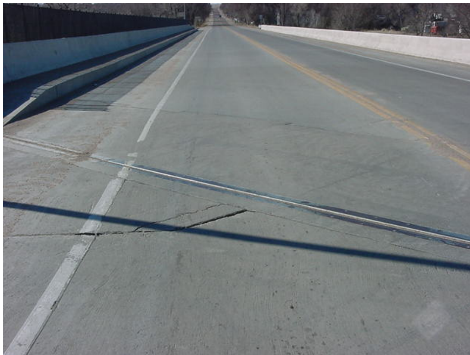
Figure C.14. Photos of Structure G-22-BX in Region 1.
