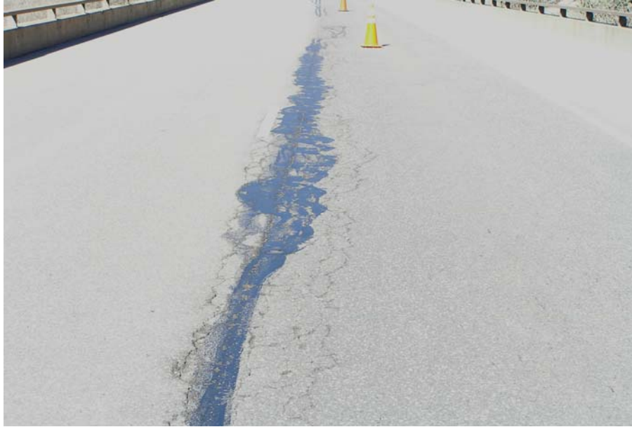
Figure 14. Alligator Cracking Developed Along Both Sides of the Construction Joint in Test Section 2.
