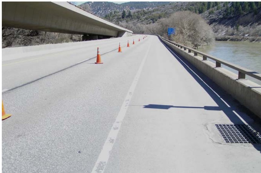
Figure 15. EB Section 3 in Excellent Condition (2005)
