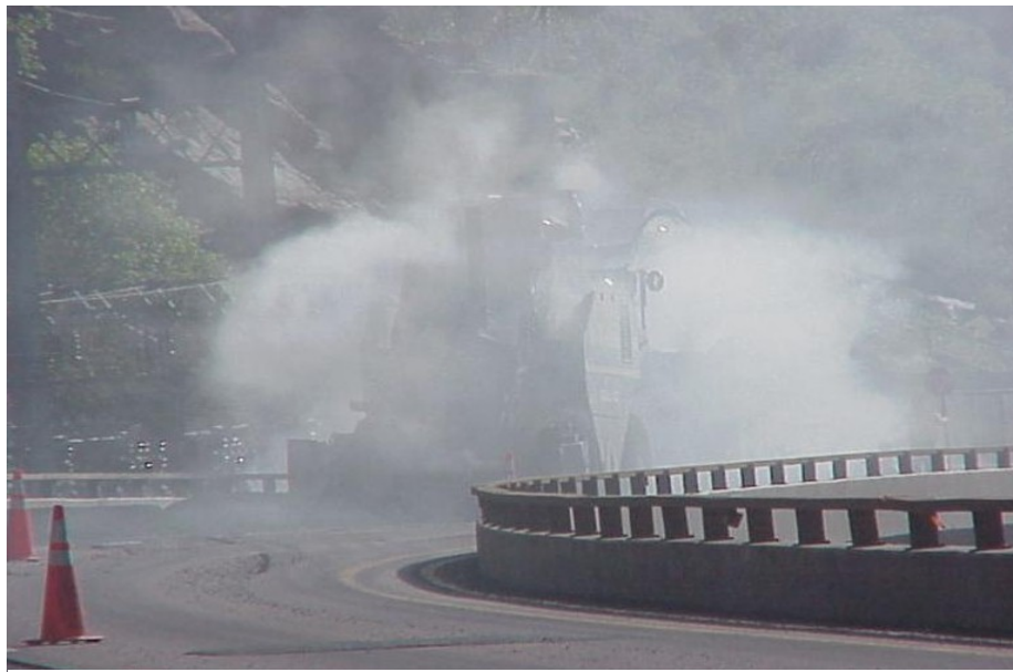
Figure 5. There Is a paver Hidden in the Smoke Behind the Transfer Vehicle. High Mix Temperatures Were Required.
