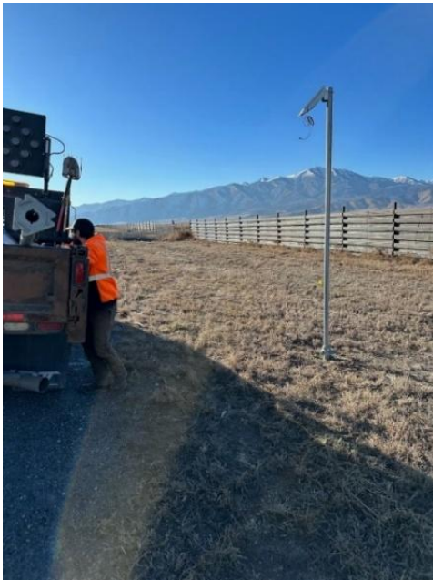
Figure 5. Posts and solar panels installed by UDOT and Stalker, left, and Stalker Traffic Data Collectors with solar panels, right. Photo credits: UDOT and P. Cramer.
