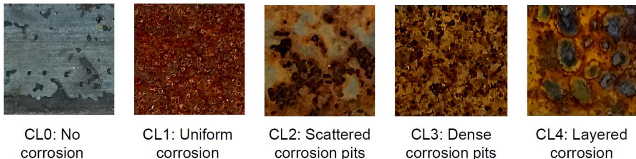
Figure 4. Surface Condition of Corroded Steel Plates. CL = corrosion level.
