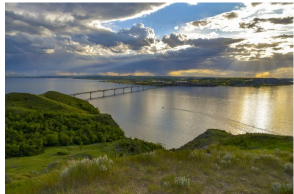
Four Bears Bridge, New Town, North Dakota (Source: North Dakota DOT)
