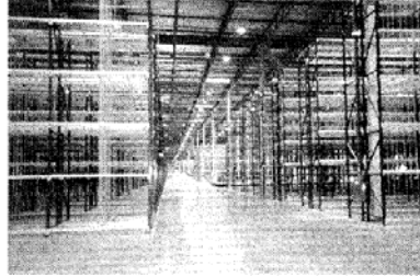
Concrete floors designed with joint spacing of 150-ft provide building owners with a very low life cycle cost floor solution.
