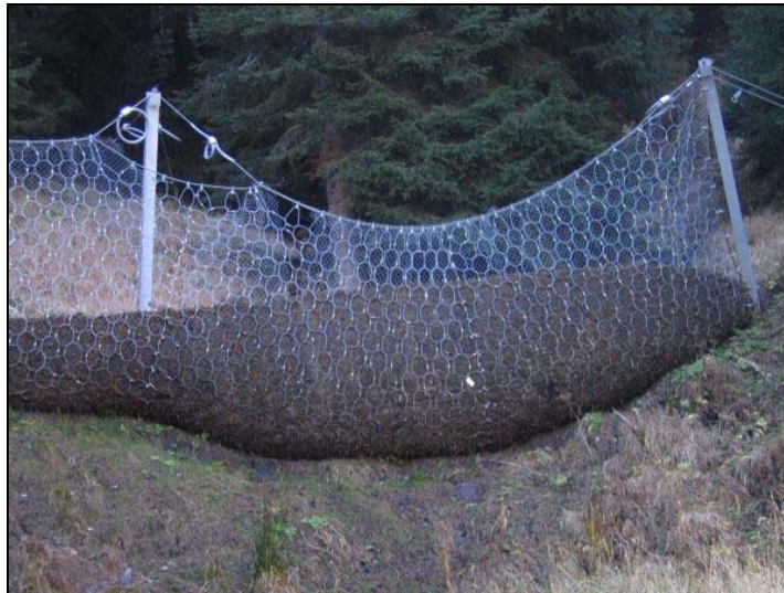
Figure 3 – The use of a high tensile-strength ring net to contain a debris flow (from www.wsl.ch )
