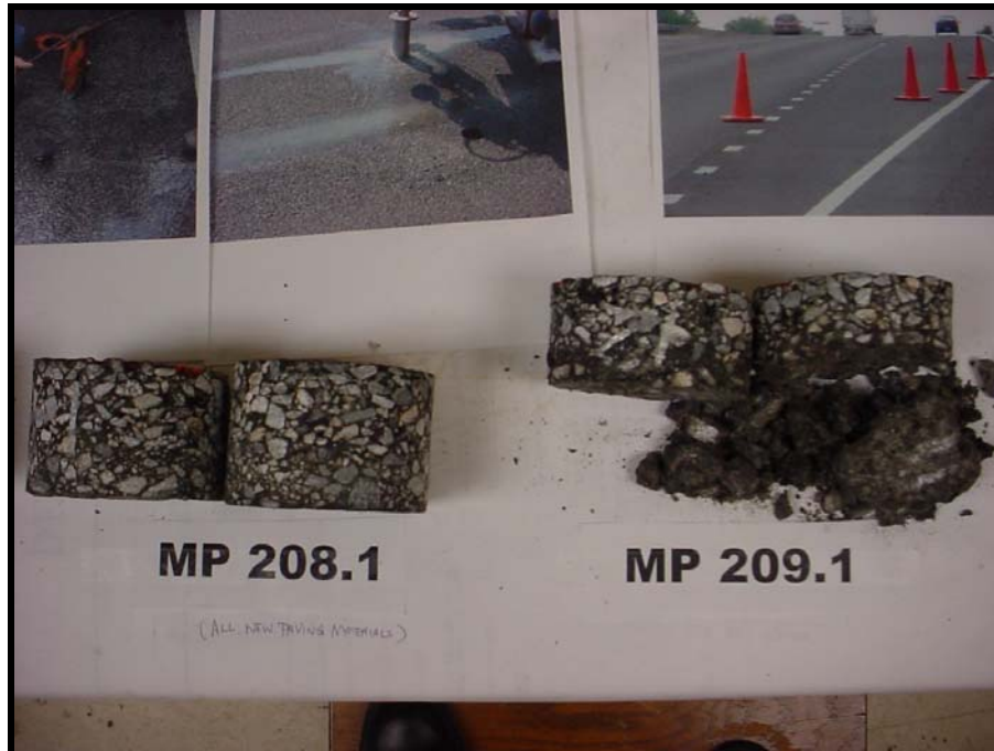
Core samples showing stripping from moisture damage
