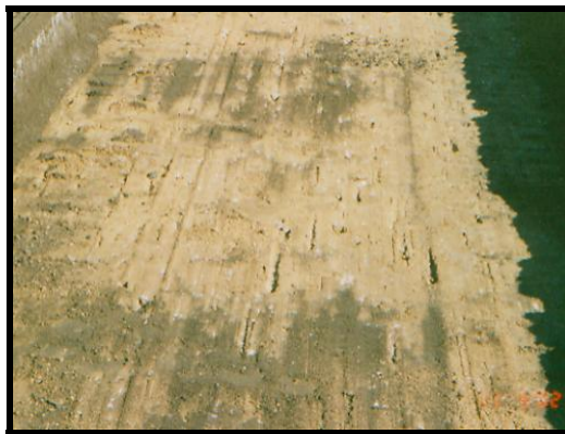
Figure 3: Roadbase exposed during asphalt remediation
