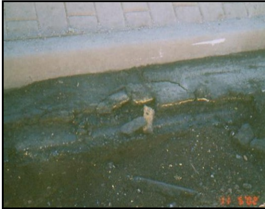
Figure 31: Asphalt removals during rehabilitation construction
