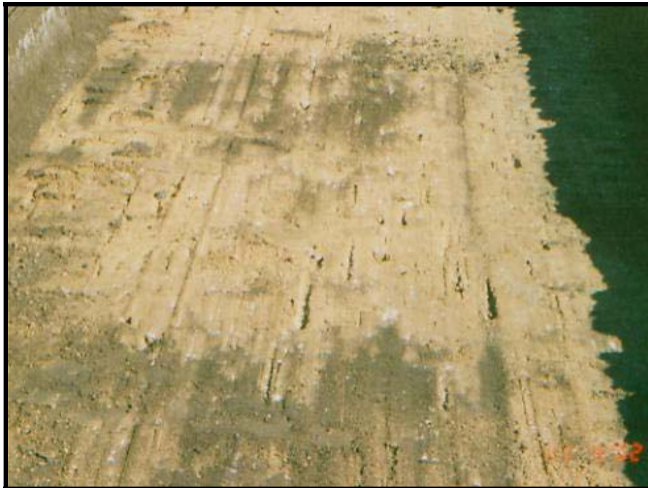
Figure 30: Roadbase exposed during remediation
