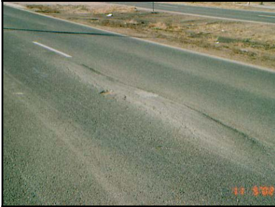
Figure 29: Failed SMA
