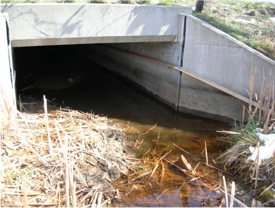
Culvert 1. Dry Creek Ditch No. 2 at U.S. 36.
