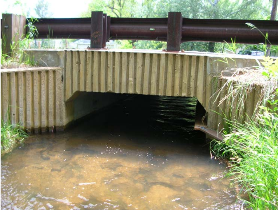
Culvert 5. Marshallville Ditch at Marshall Road. Both ledge and ramp visible at right; note strap hinge to connect them.
