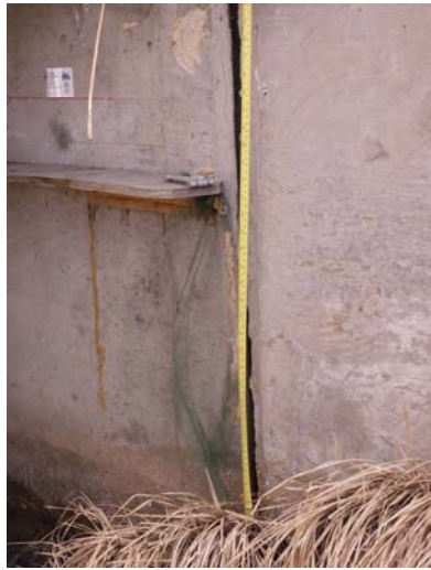
End of ledge at Dry Creek No. 2 Ditch culvert at U.S. 36. Note hinge to connect ramp. Distance from ledge to ground is 54 cm. Bird netting is visible.
