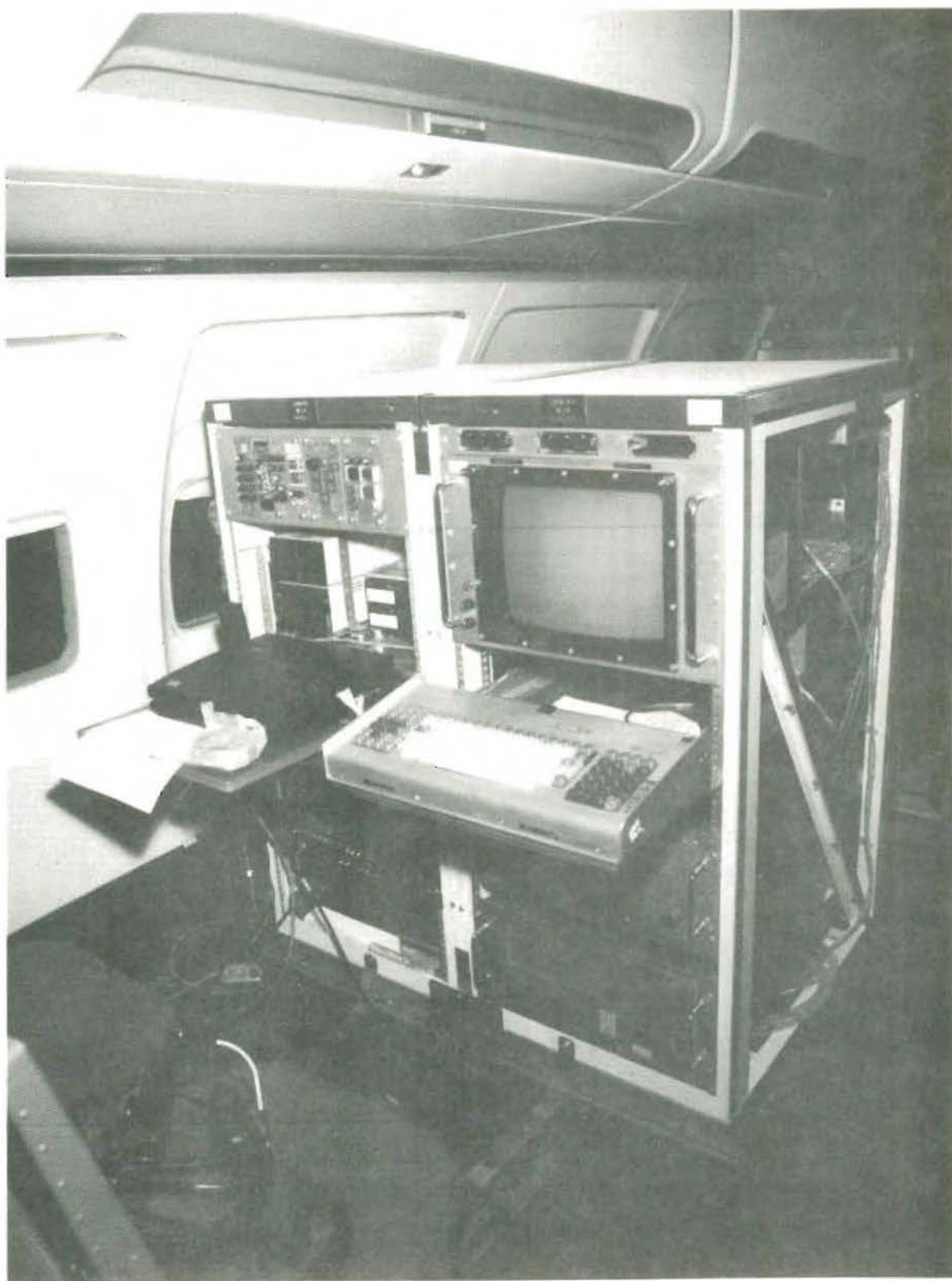
FIGURE 2.1.1-8 INSTRUMENT RACK, STATION 1548, LEFT SIDE
