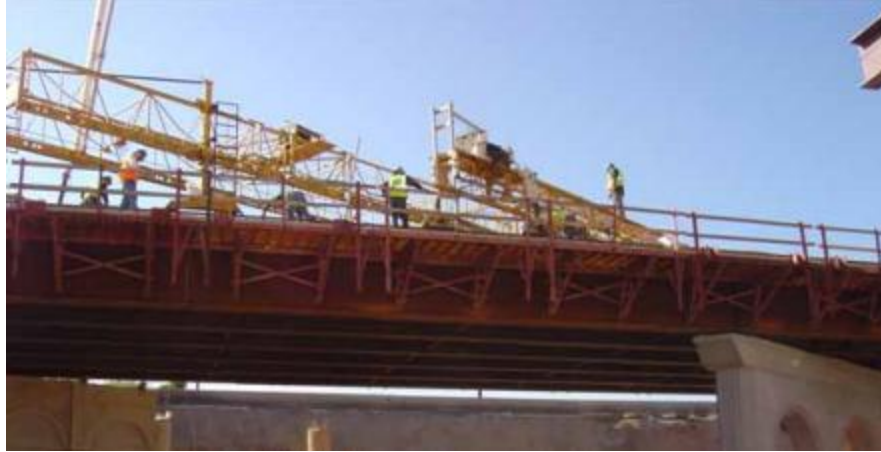
Figure 4-16. Lubbock Bridge During Deck Pour (Romage, 2008)
