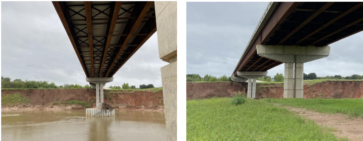
Figure 3-7. SH 105 Bridge Span 7-8
