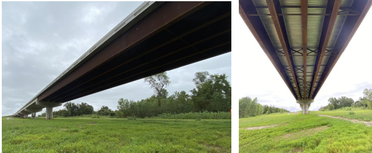
Figure 3-8. SH 105 Bridge Span 6
