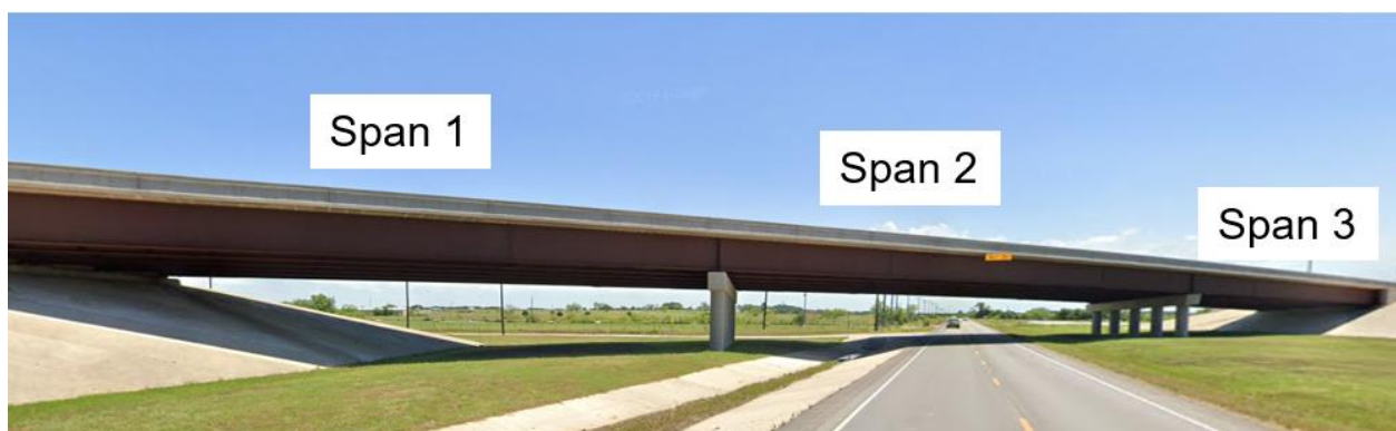
Figure 3-21. Chisholm Trail Bridge Spans
