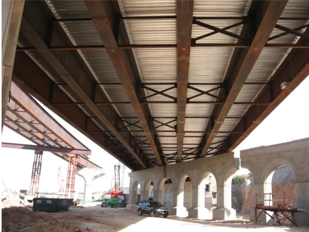
Figure 2-9. Lean-on Bracing in Lubbock Texas Implementation Study (TxDOT Project 5-1772)
