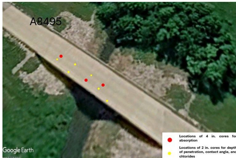
Figure 6.4. Aerial photograph for bridge A8495 and the core locations
