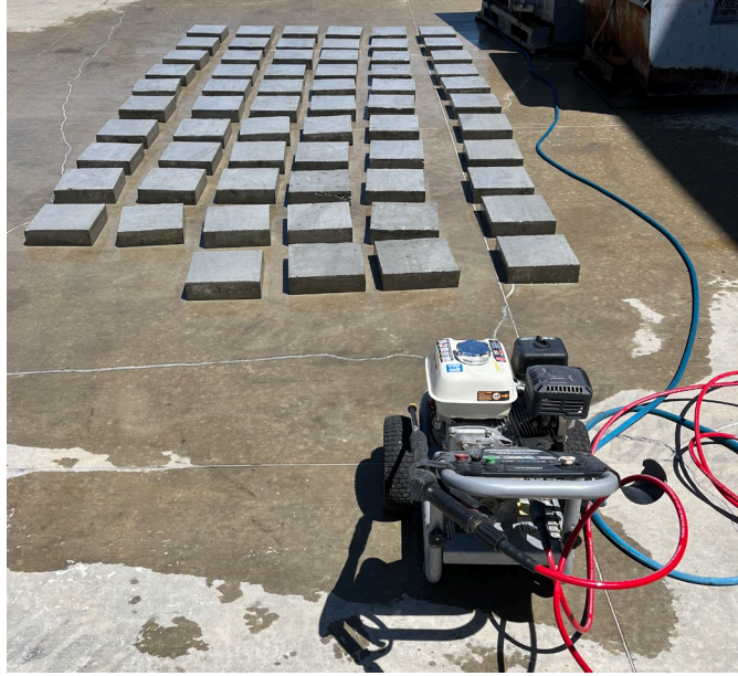
Figure 4.1. Concrete surface preparation by hydro-jetting
