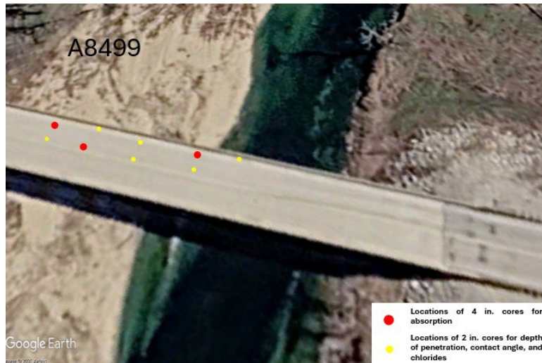
Figure 6.5. Aerial photograph for bridge A8499 and core locations
