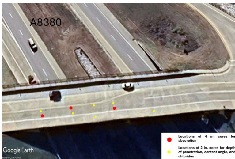
Figure 6.2. Aerial photograph for bridge A8380 and the core locations
