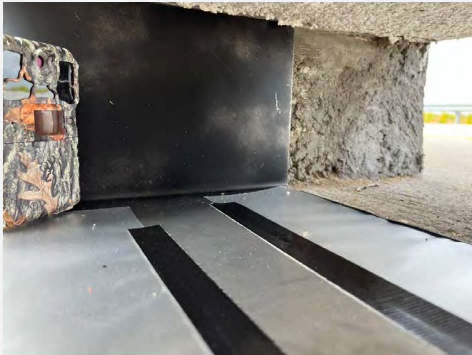
Photo 1. Camera/track plate installed in scupper. Tracking medium in middle with contact paper on sides.
