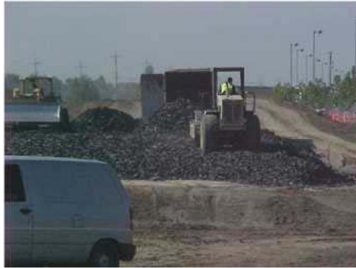
Caltrans uses shredded tires in highway embankments
