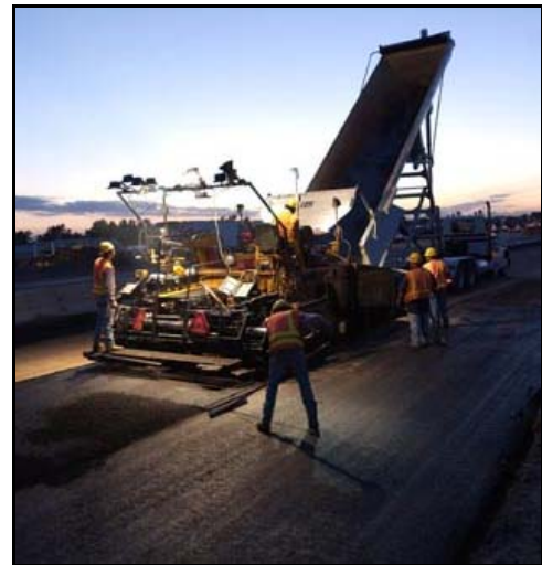
Figure 1. Asphalt Paving Operations on the T-REX Project
