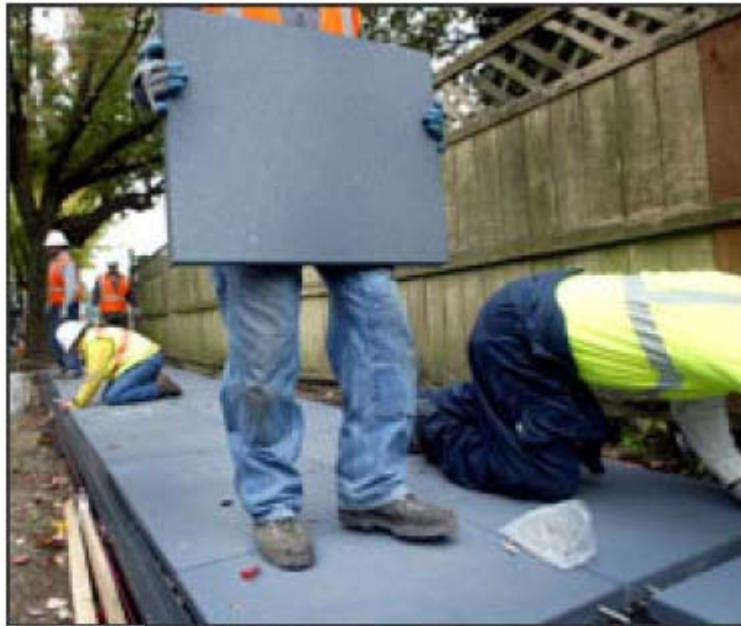
Figure F-4 Rubber Sidewalk Installation
