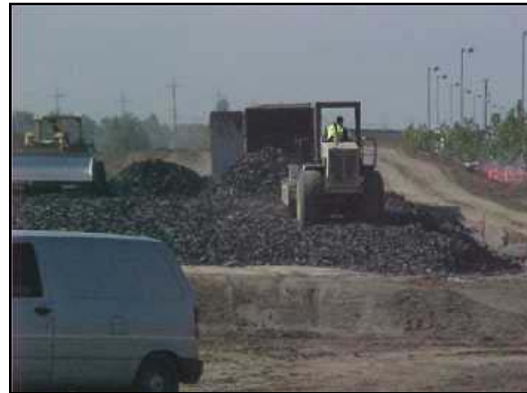
Figure 4. Caltrans Uses Shredded Tires in Highway Embankments
