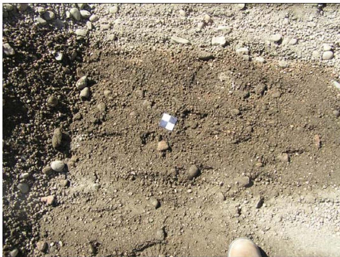
Figure 4. Mt. Vernon Canyon's 1/2" pea gravel arrester bed is heavily polluted by fine material. A quantity of 1" aggregate was added to the bed at some time.
