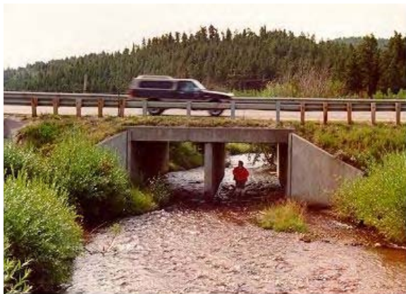
Control Site 1: Deer Creek span bridge 1
