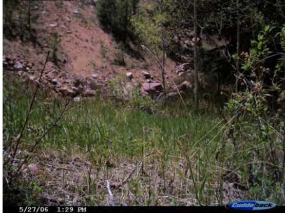
Impact Site 1: fill slope, west side
