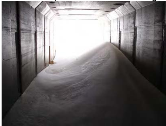
March 2006 (snow drift inside looking west)
