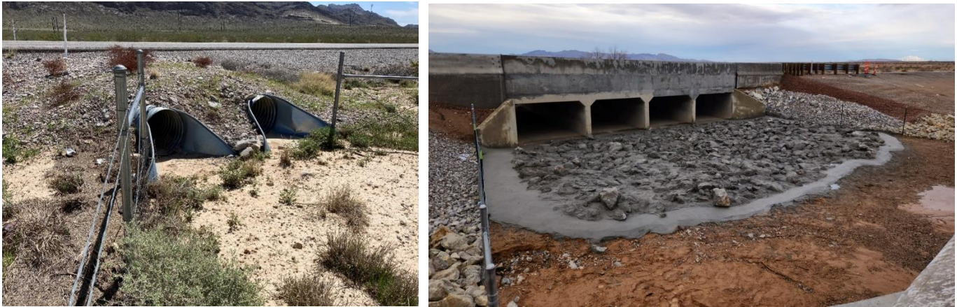
Figures 5.2 –Project Tortoise Fencing at Culverts (photos by NDOT)
