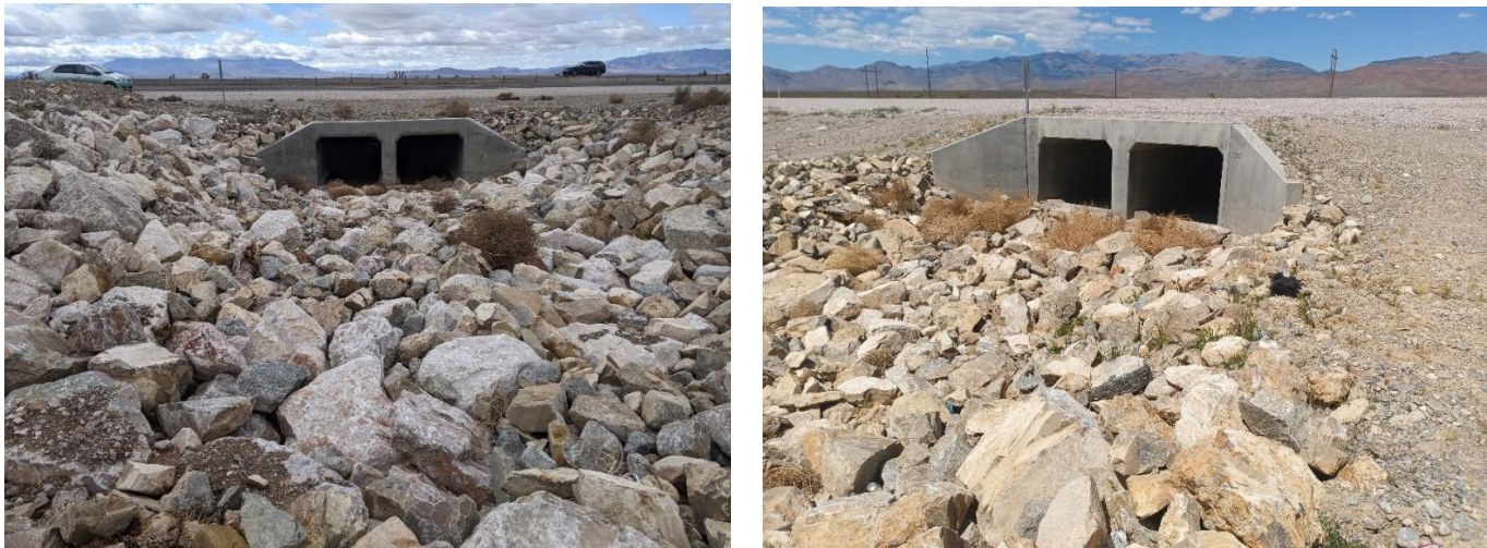
Figures 2.4 - Site D/Culvert 35 Photos—Culvert Inlet (Left) and Culvert Outfall (Right)
