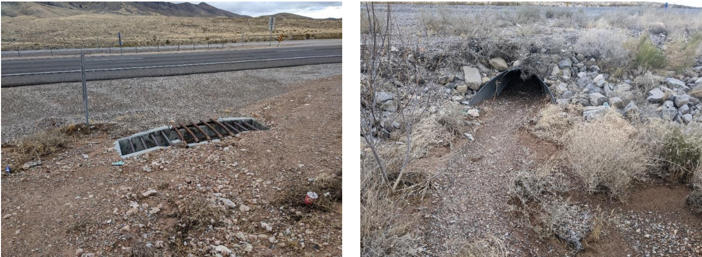
Figures 2.1 - Site A/Culvert 8 Photos—DI at Upstream End (Left) and Culvert Outfall (Right)
