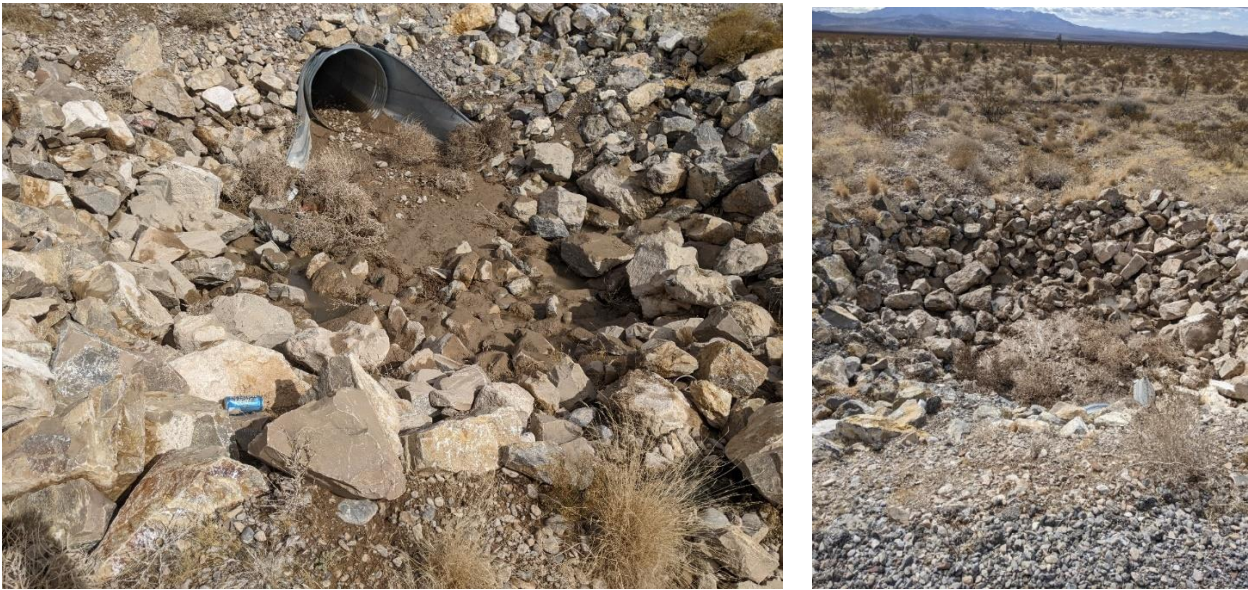
Figures 2.3 - Site C/Culvert 20 Photos—Existing Riprap Basin at Culvert Outfall
