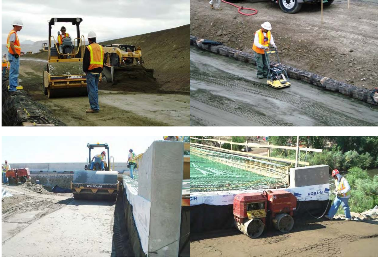
Figure 4-6. Near Wall Compaction Techniques
