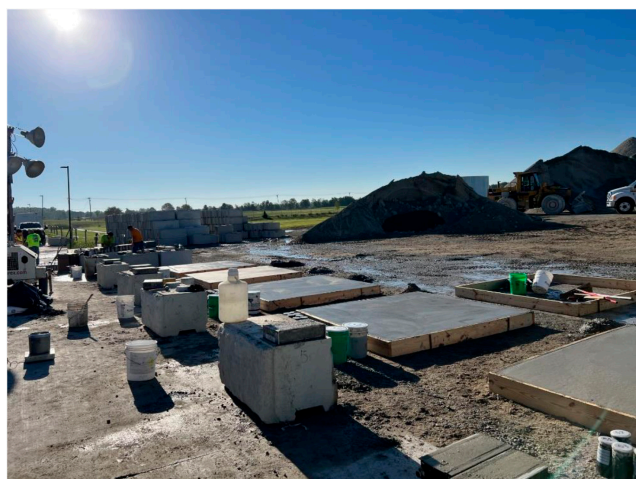
Figure 3.2 Freshly Cast Concrete Slabs Immediately After Finishing.
