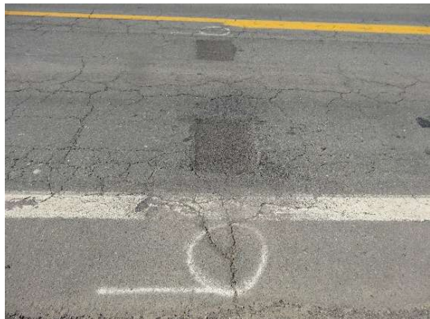
(b) Final Inspection
