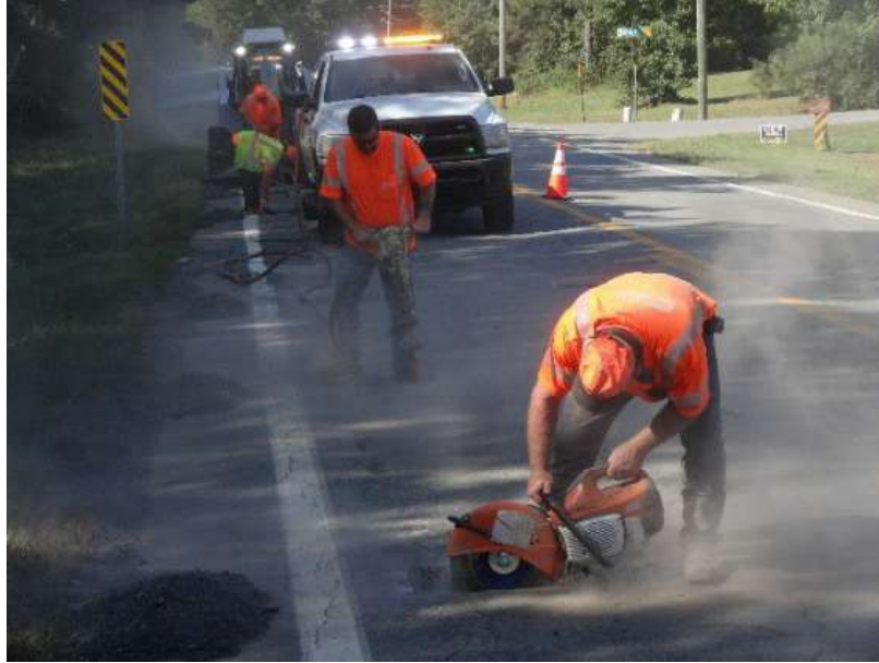
Figure 5: Cutting Edges with a Saw and Breaking with a Jackhammer
