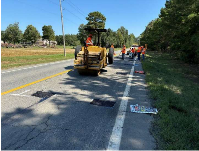
Figure 11. Compacting Placed HPCM Material
