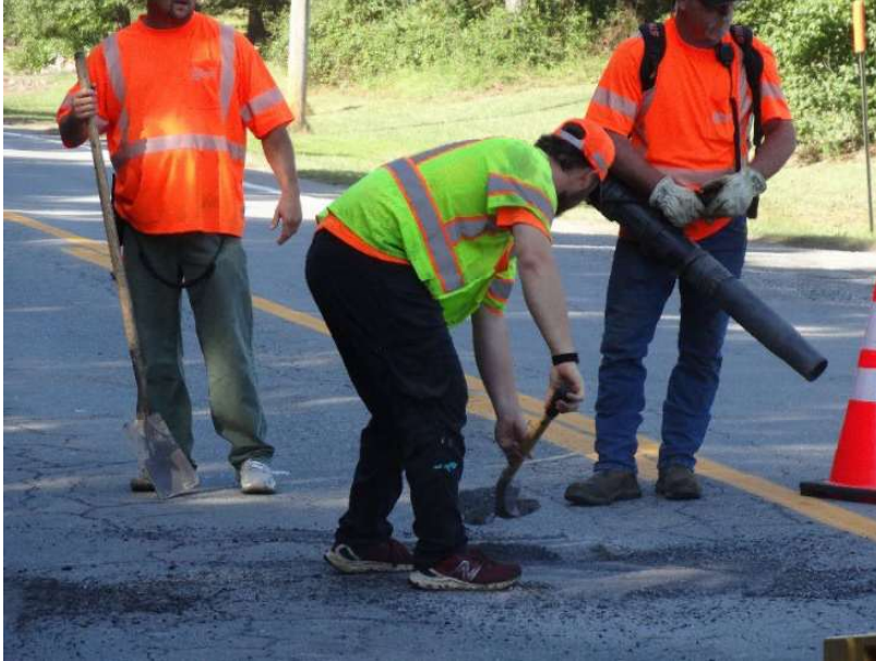
Figure 9. Placing HPCM Material in Potholes
