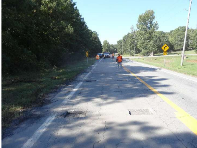
Figure 7. Prepared Site with Potholes
