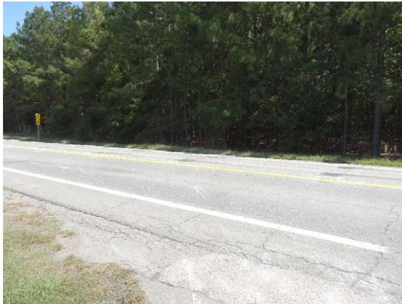
Figure 1. Highway 338, Dixon Road, Little Rock, Arkansas
