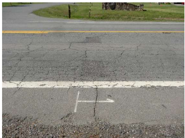
(b) Final Inspection
