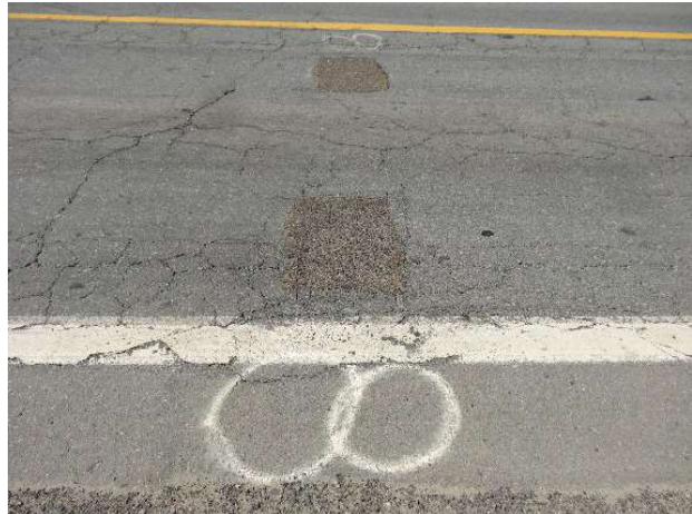
(b) Final Inspection
