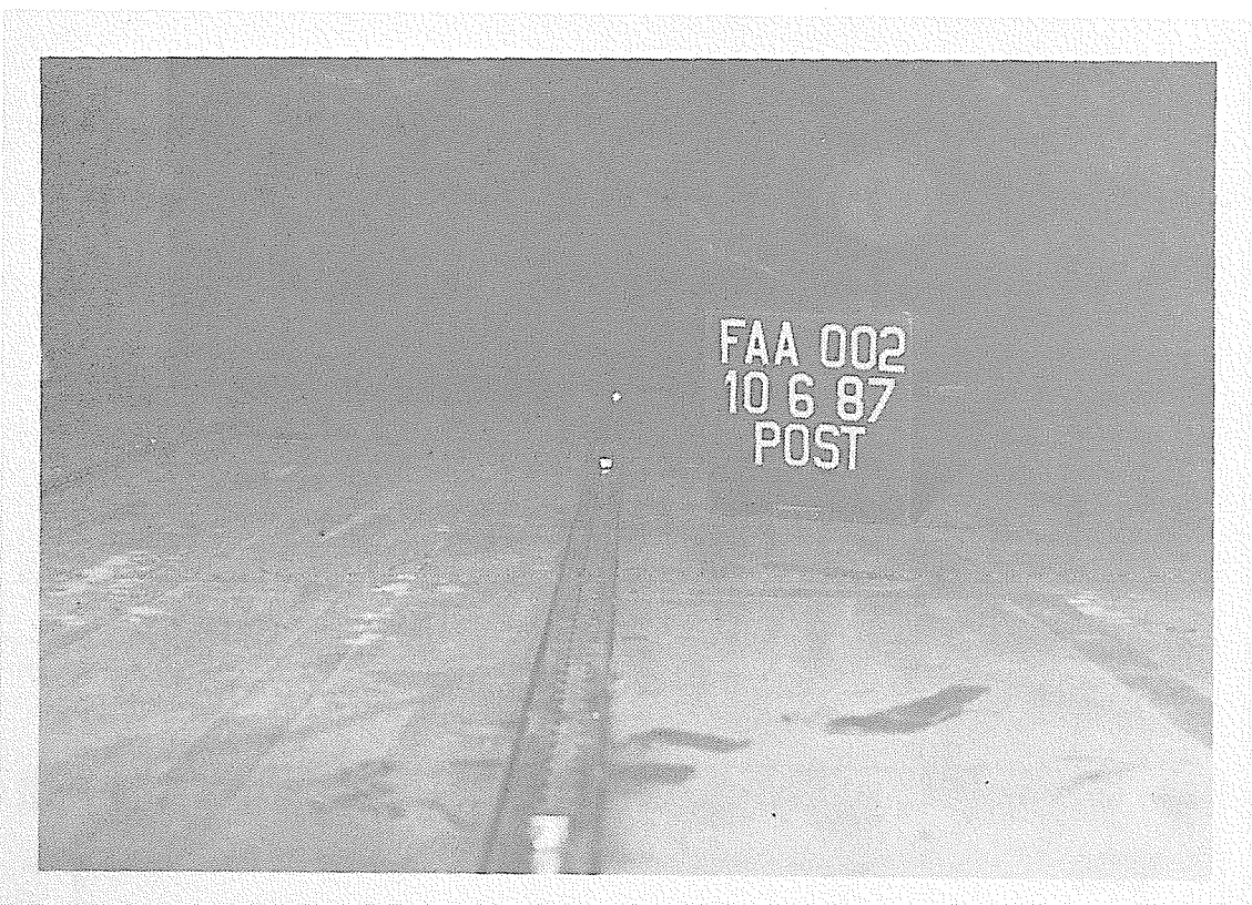
Figure 50. POST-TEST 02 FLOOR - VIEW 3
