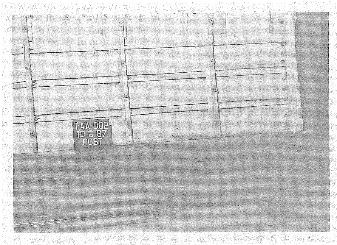
Figure 51. POST-TEST 02 FLOOR - VIEW 4
