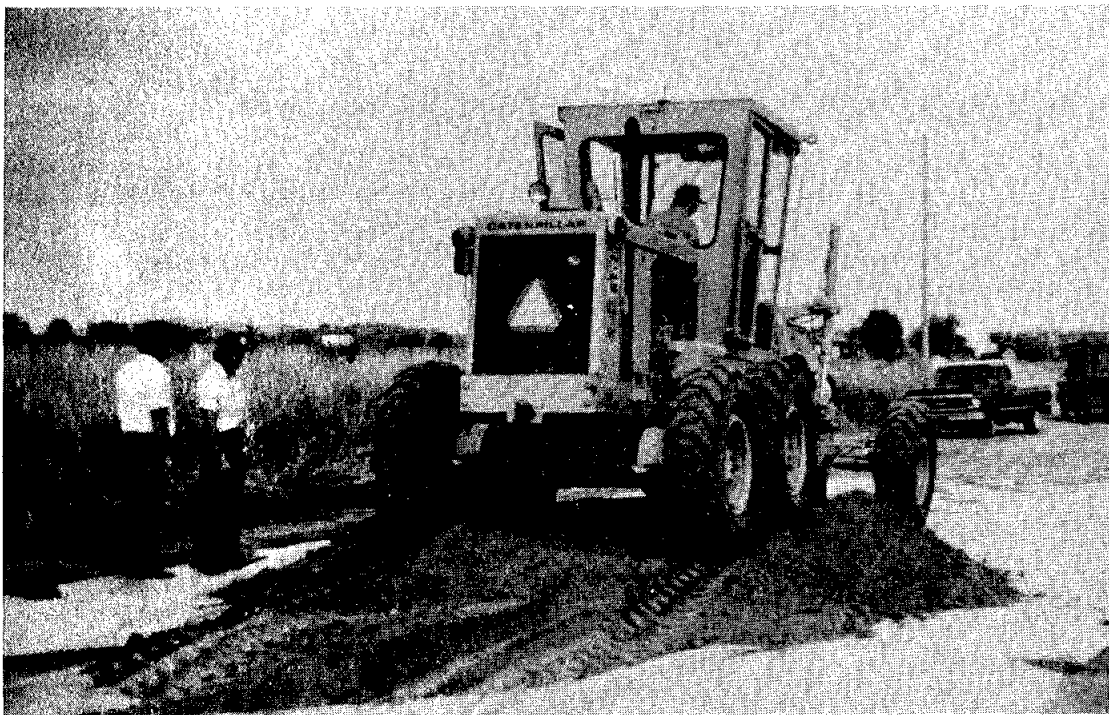
FIGURE 6.8 BLADING MOUNDS FROM TRAILER DUMP
