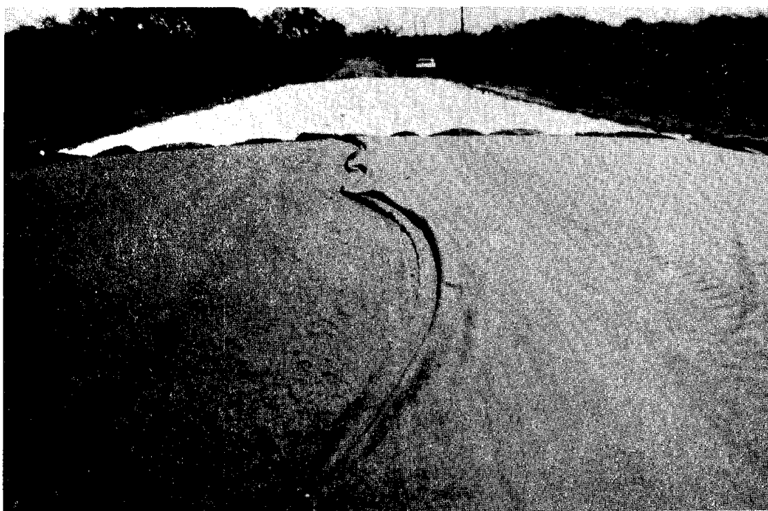
FIGURE 4.12 CENTER LAP BLOWN APART
