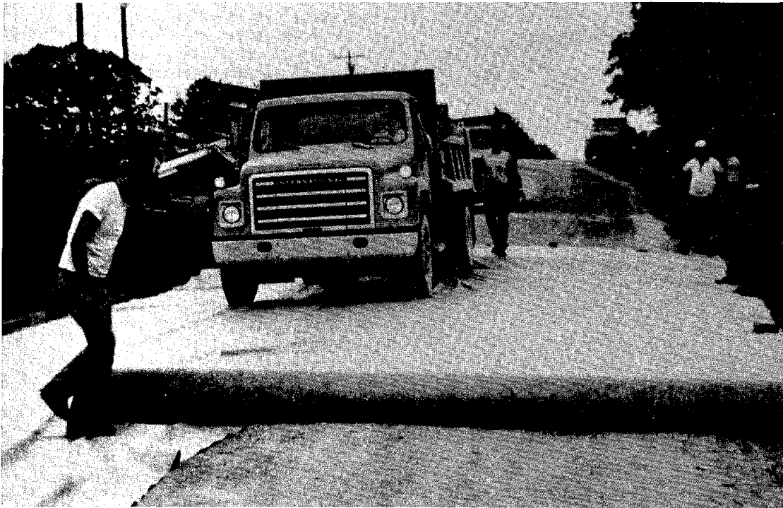
FIGURE 5.8 DUMPING 5 FEET FROM STARTING END
