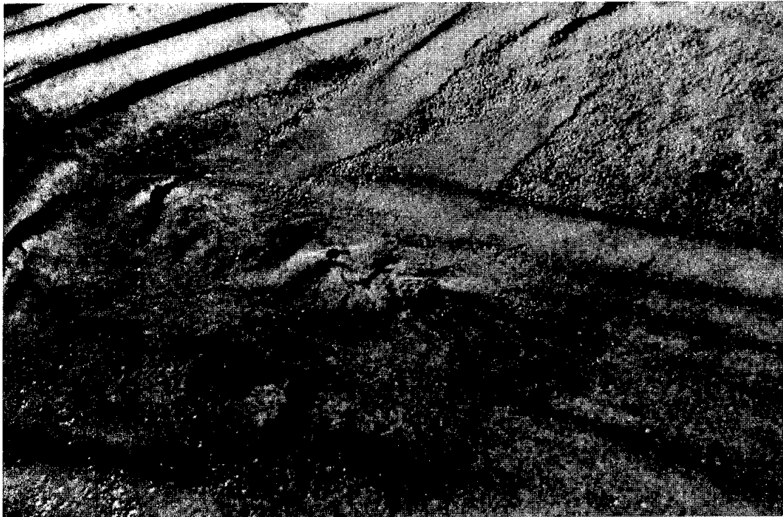
FIGURE 4.16 LARGE FOLDS CREATING PROBLEMS
