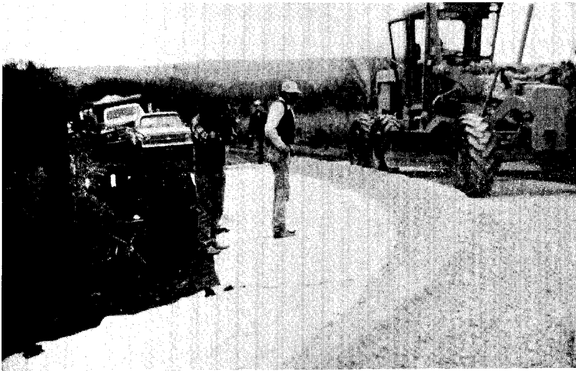
FIGURE 4.17 FABRIC INSTALLATION ON CURVE
