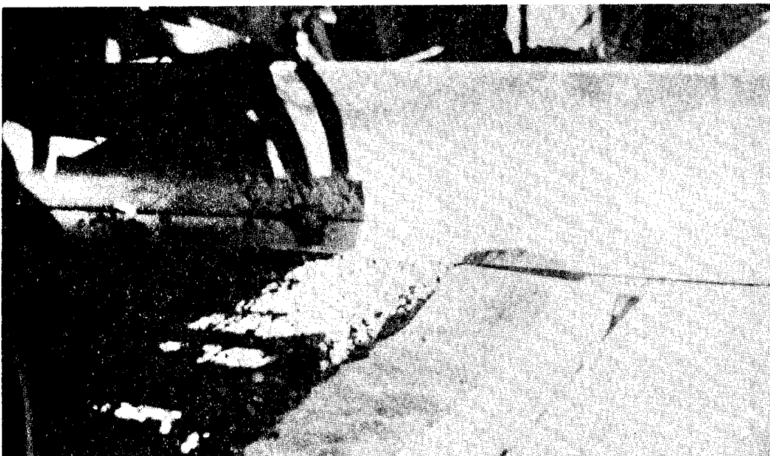
FIGURE 6.2 BLADE TOO CLOSE TO FABRIC
