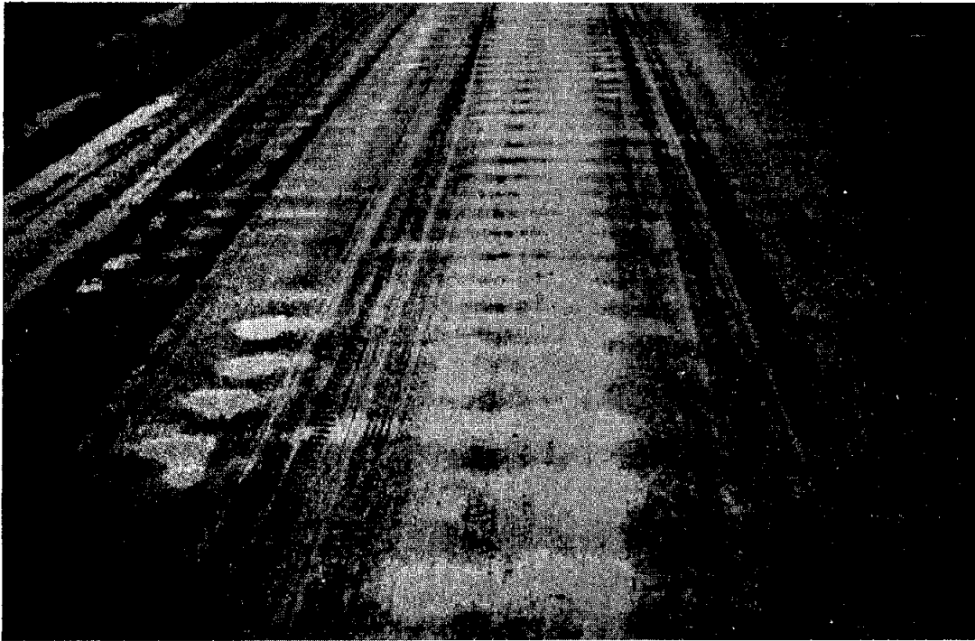
FIGURE 2.6 GRANULAR ROAD ( WASHBOARDING )
