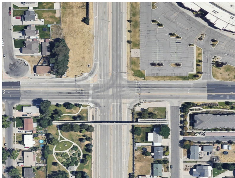
Figure 7: Aerial view of the continuous flow intersection (CFI) at Bangerter Highway and 3100 South
