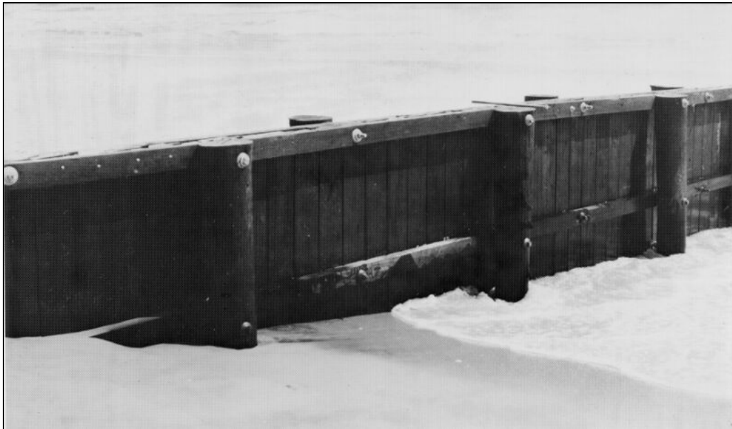
Figure 7.16. Timber pile groin.
