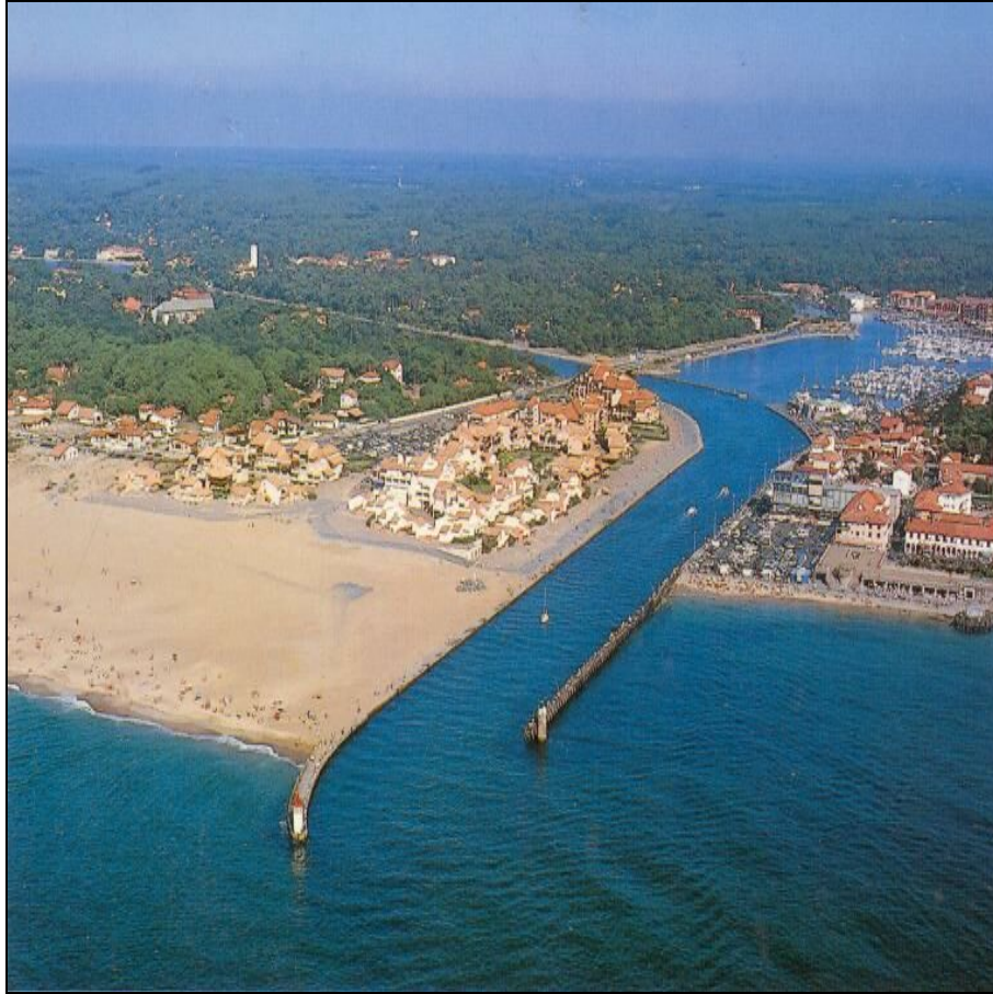
Figure 7.12. Jetty entrance for navigation channel. (Note the updrift sediment and starved downdrift shoreline.)
