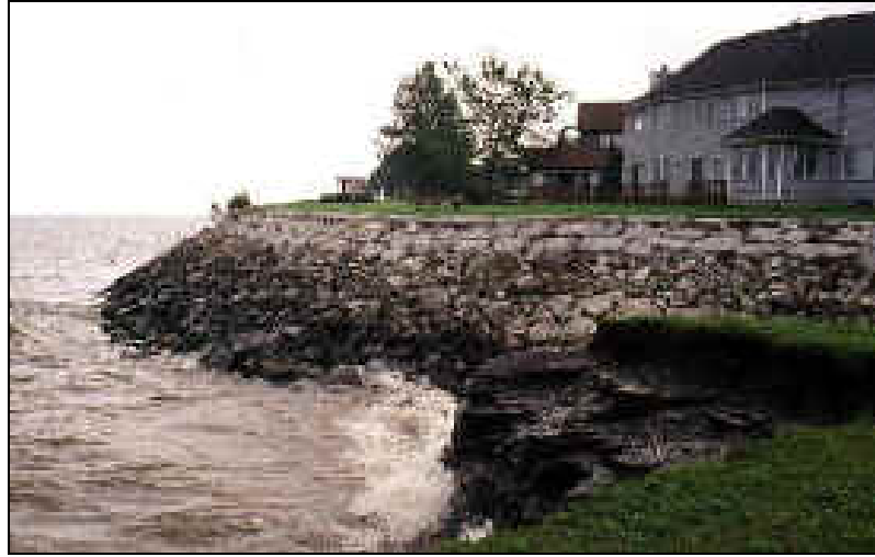
Figure 7.10. Stone revetment.
