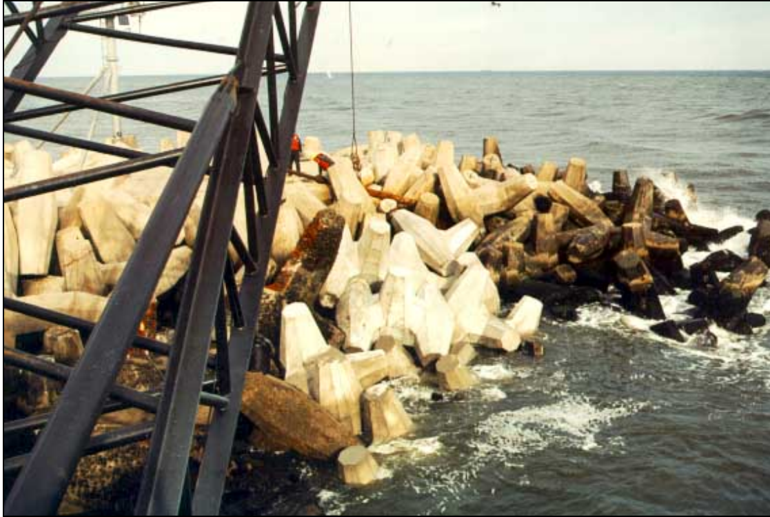
Figure 7.13. Core-loc Armor Units on Manasquan Jetties being placed over dolos. (The darker units are dolos.)
