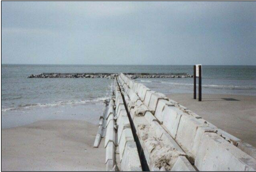
Figure 7.15. Concrete groin constructed with precast units. (Note the stone protection around the "T" at the seaward end.)
