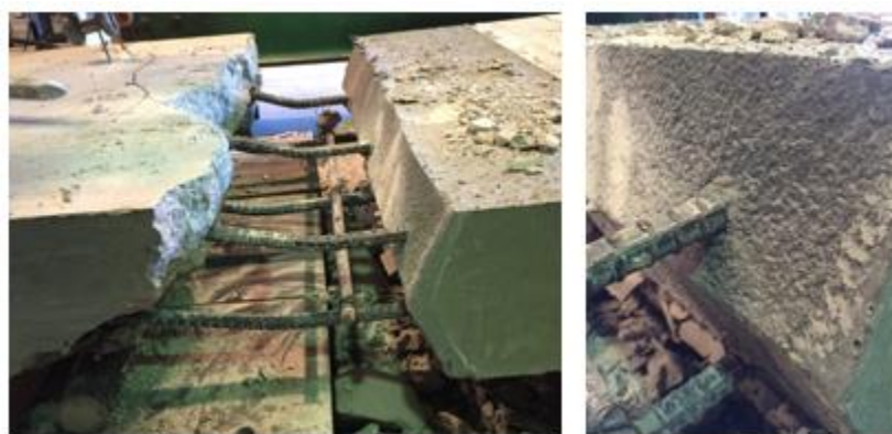
Figure 15. Longitudinal connection joint investigation
