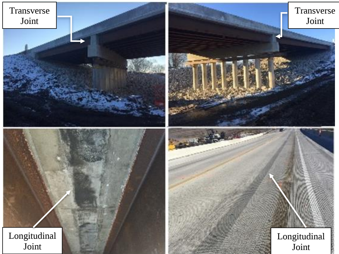
Figure 4. Constructed Little Silver Creek Bridge
