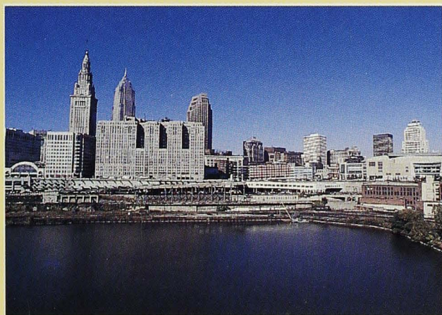
Greater Cleveland Passenger Accessway Cleveland, Ohio
