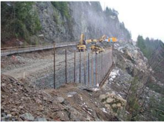
Figure 1.1: Road construction in steep slope
