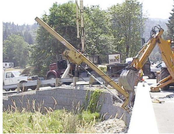
Figure 1.2: Micropile installation equipment
