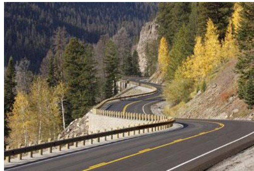
Figure 1.3: A finished roadway in mountainous areas
