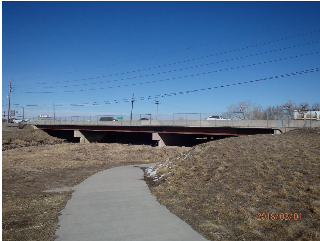
Figure 2. Photo of Structure E-16-P
