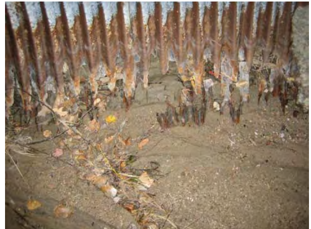
Figure 7. Culvert pipe corrosion near Castle Rock, I-25
