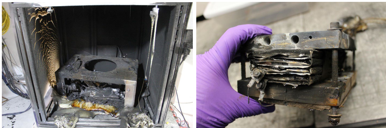
Figure 12. Post-overtemperature images of the 4p2s LFP/graphite battery pack
