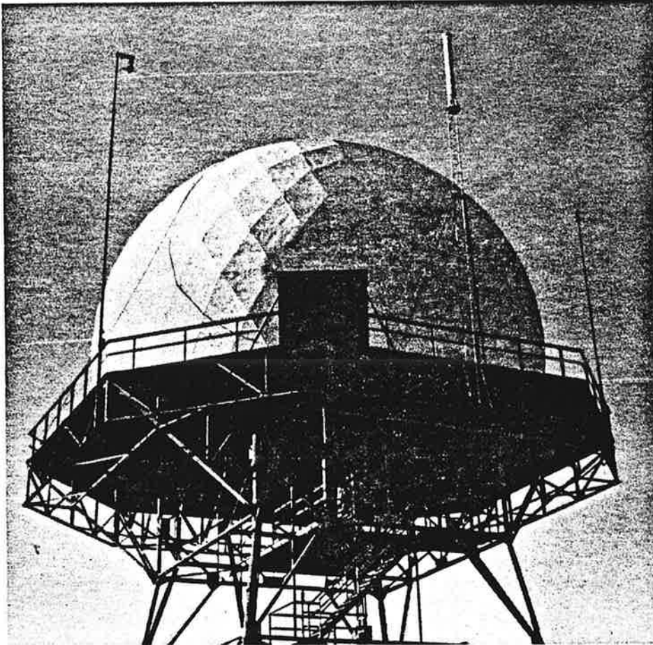
Figure 4-2. ARSR Omni Installation at Elwood, New Jersey
