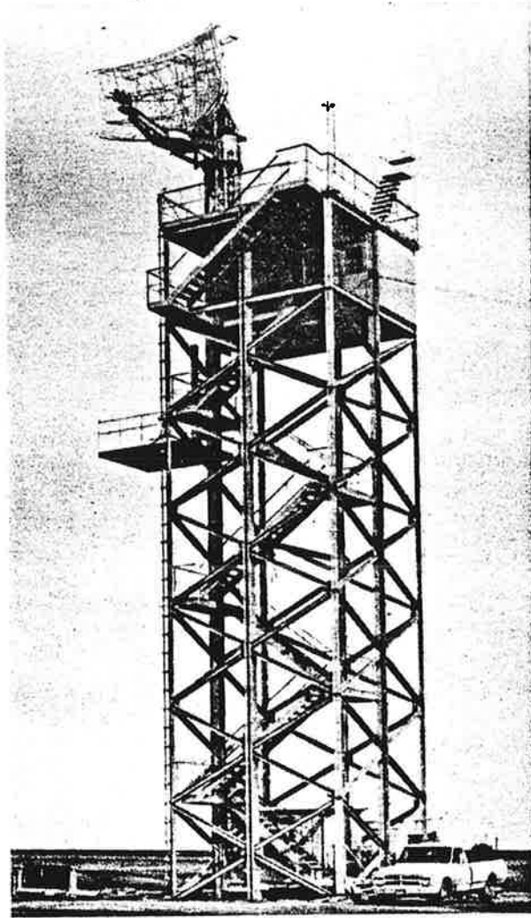
Figure 2-13. Antenna Test Tower
