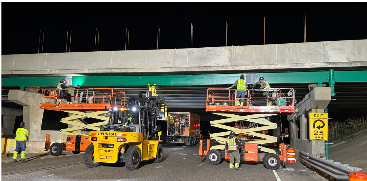
Figure 7. Photo. Installation of a “zipper detail” repair for IDOT bridge SN 084-0077 Girder 19 (fascia girder). The replacement section has been lifted into place, but bolts have not yet been installed.
