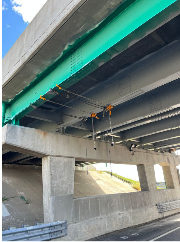
Figure 6. Photo. Straightening IDOT bridge SN 084-0077 Girder 10 (fascia girder) using chains attached to Girder 11 (first interior girder).
