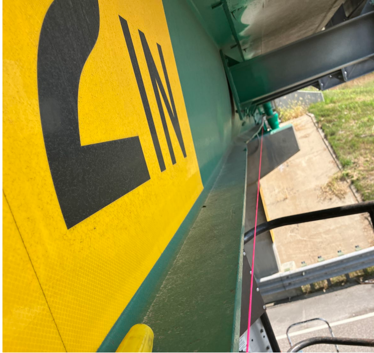
Figure 4. Photo. Stringline placement for hand measurements of flange deflections on IDOT bridge SN 084-0077 Girder 19. (The stringline is colored pink.)
