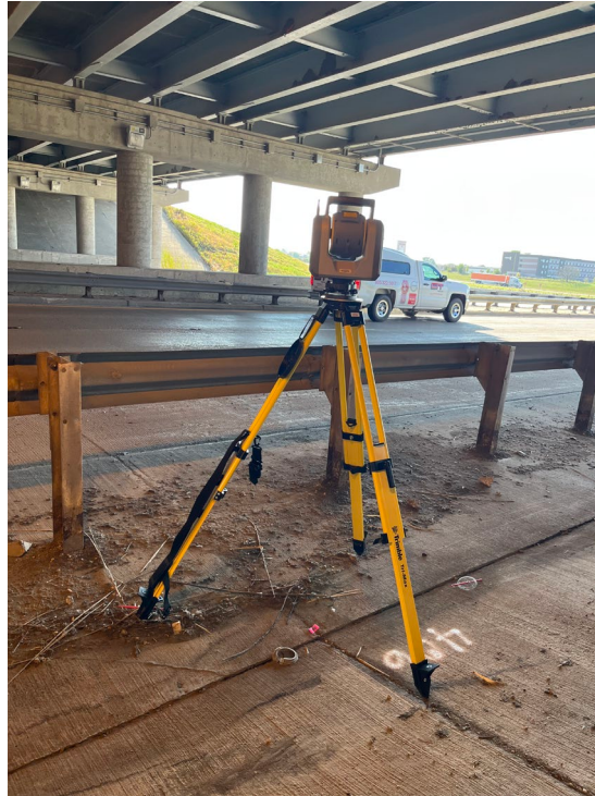
C. Scanner positioned on the shoulder underneath a bridge.
