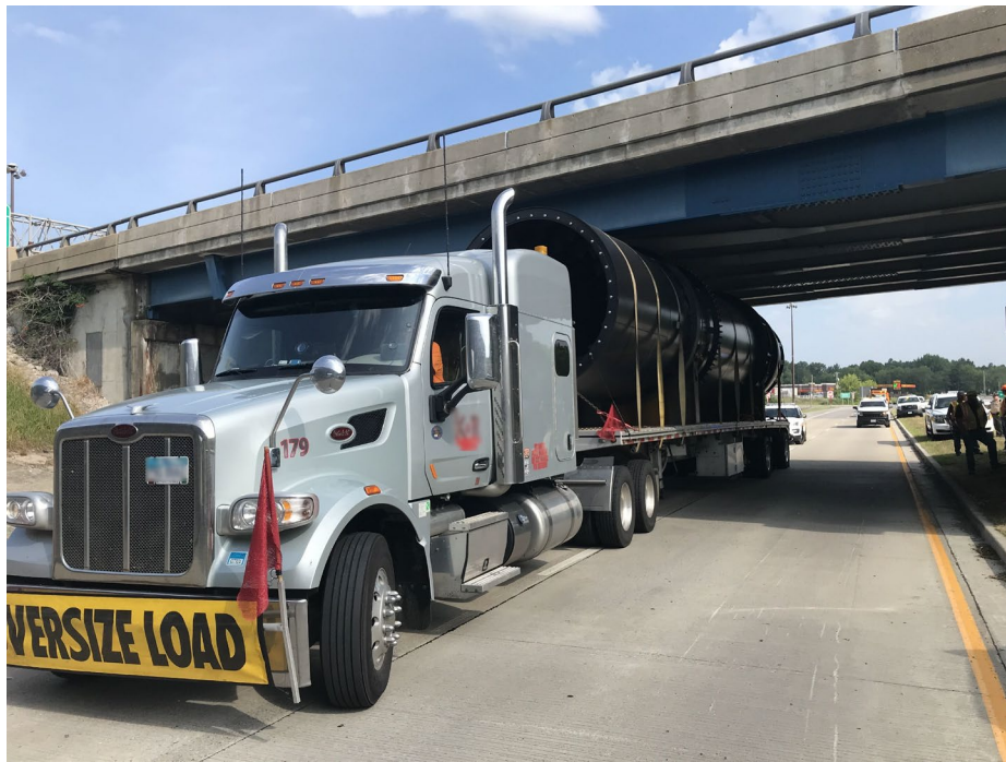
Figure 1. Photo. Over-height vehicle lodged beneath a bridge following an impact incident.
