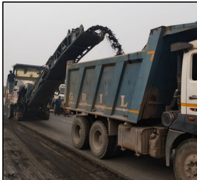
Figure 2.2. Milling of asphalt pavement
