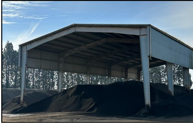
Figure 2.7. Roofing of RAP material for minimizing moisture concerns
