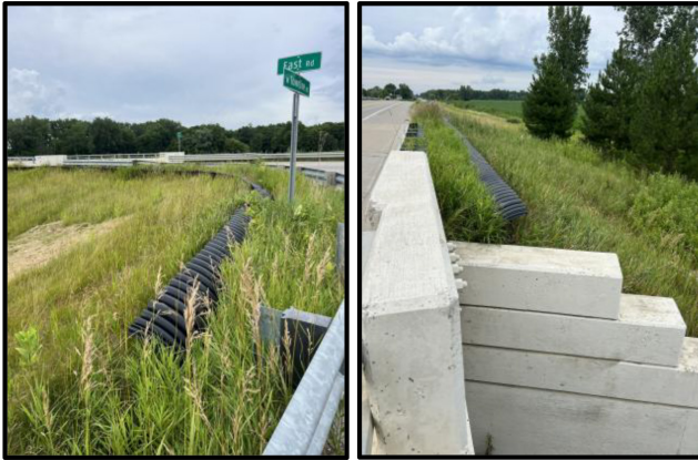
Figure 5.4 Snake Barrier Made from 36-in. Corrugated Pipe.
