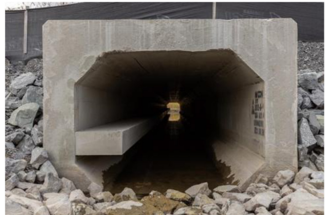
Figure 7.1 Box Culvert for Amphibian Crossing. Source: MCON (n.d.).
