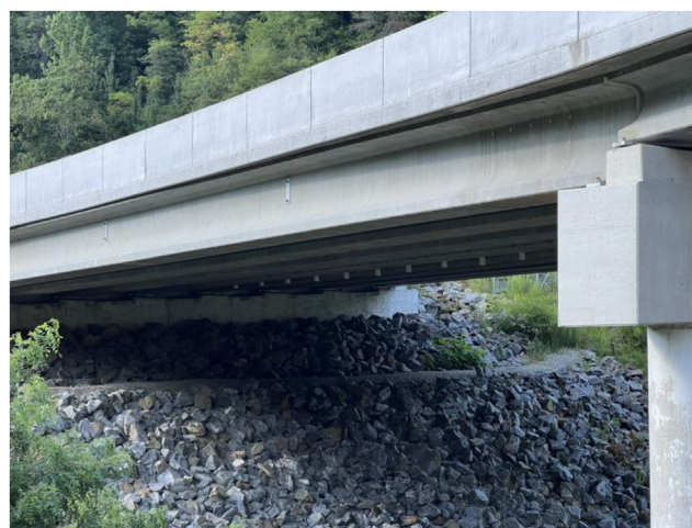
Figure 5.12 Flat Gravel Path Under Road for Larger Mammals.
