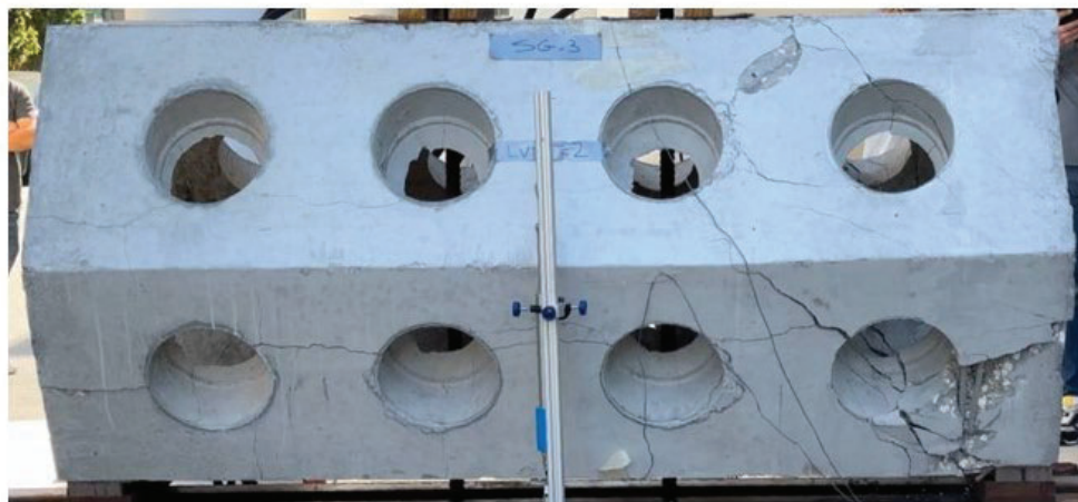
Figure 13 Cracking pattern of FB-2 near the end of the final cycle
