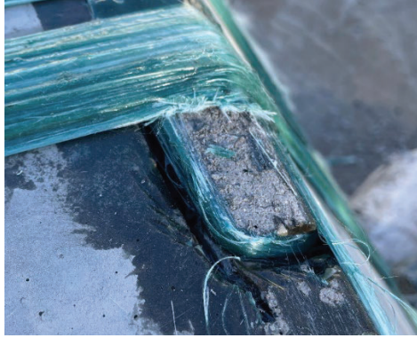
Figure 27 Anchoring fibers on both ends of the longitudinal strips for FS-2
