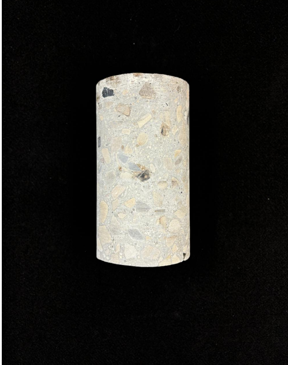
Figure D.19 Core 4 of normal-weight concrete approach slabs at bridge C-989.
