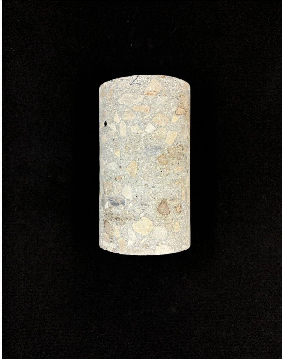
Figure D.17 Core 2 of normal-weight concrete approach slabs at bridge C-989.
