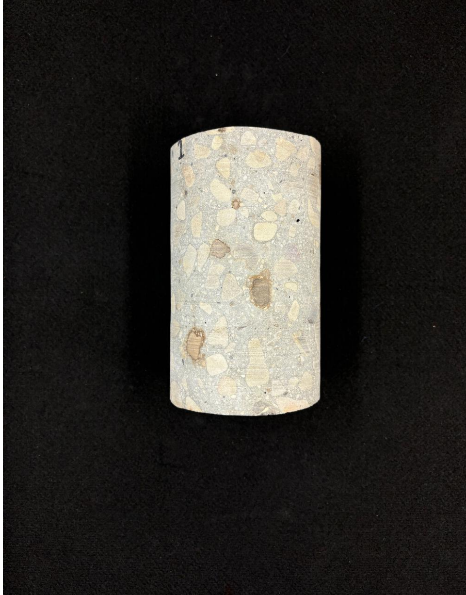
Figure D.16 Core 1 of normal-weight concrete approach slabs at bridge C-989.
