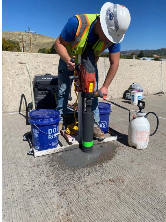
Figure 3.7 Coring machine.
