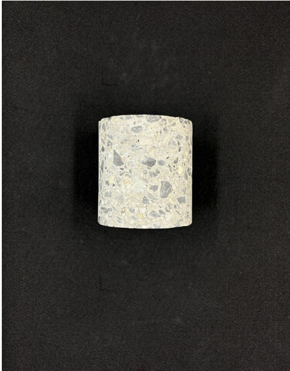
Figure D.12 Core 2 of lightweight concrete deck at bridge F-792.
