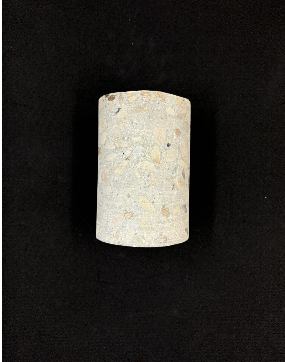
Figure D.20 Core 5 of normal-weight concrete approach slabs at bridge C-989.
