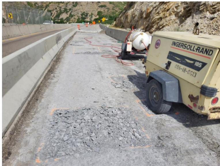
Figure 1.2 Emergency repair of lightweight concrete bridge deck.
