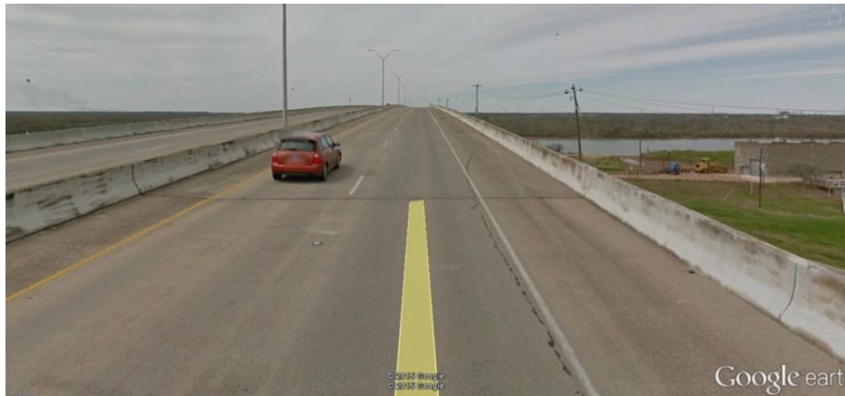
Exhibit 5-3: SH 36 Bridge over the Brazos River
