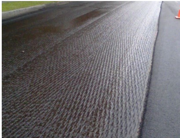
Figure 66. Uniform Application of Tack Coat
