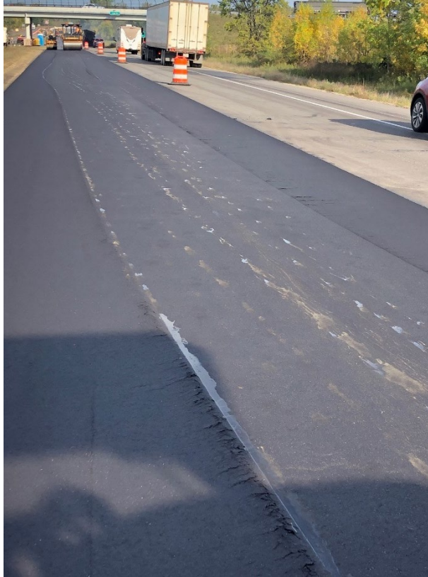
Figure 174. Roller Marks in a Freshly Laid Asphalt Pavement
