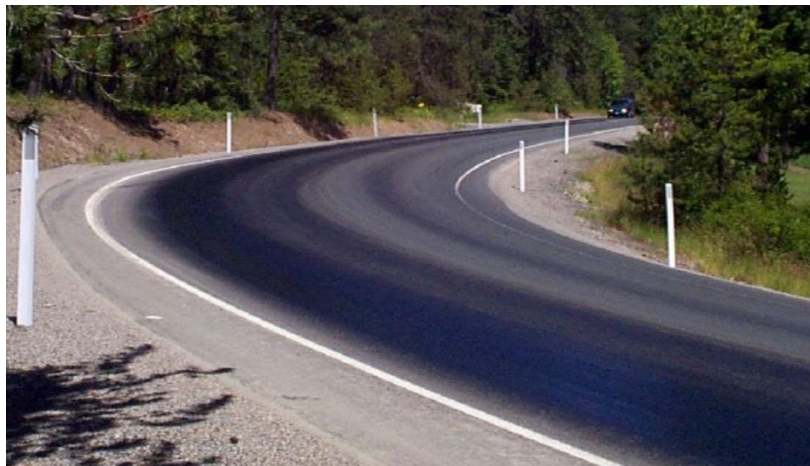
Figure 171. Asphalt Bleeding in the Travel Lane
