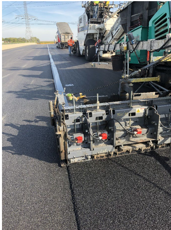
Figure 92. Fixed-Width Screed with Vibratory Bolt-On Extensions
