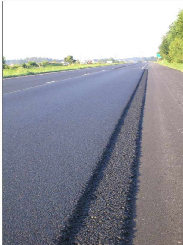
Figure 133. Notched-Wedge Joint with Taper at Top and Bottom of Wedge
