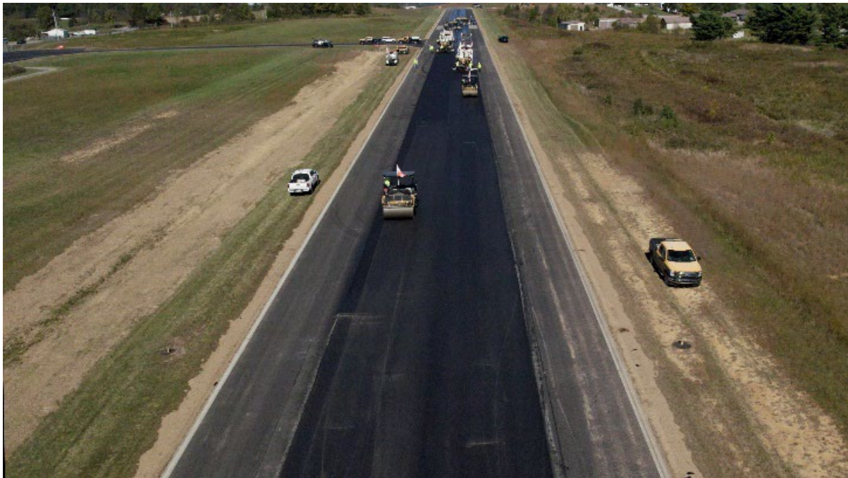
Figure 123. Longitudinal Joints on Airfield Runway
