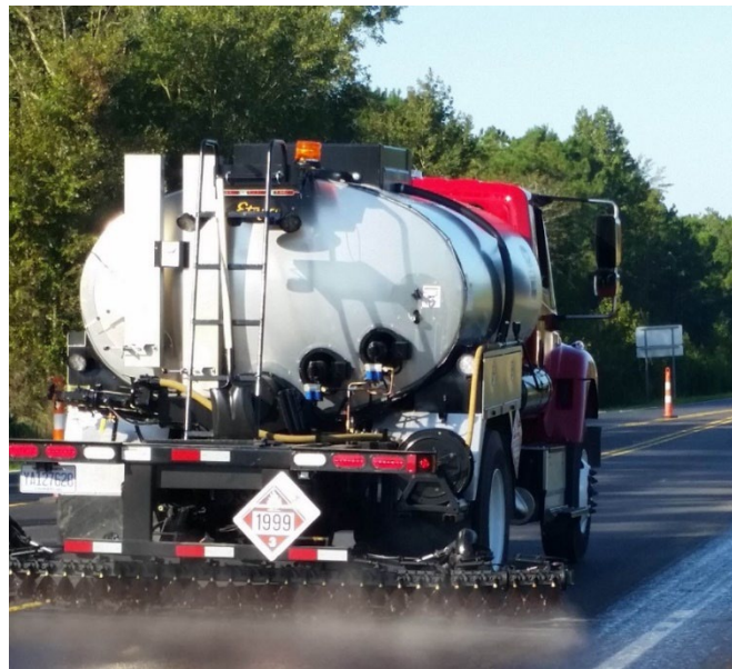
Figure 63. Distributor Applying Tack Coat
