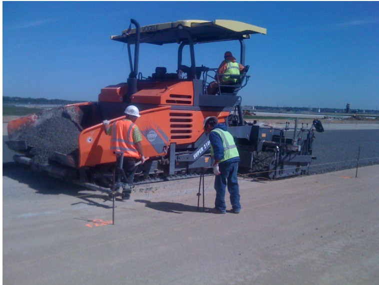
Figure 105. Stringline on an Airfield Project
