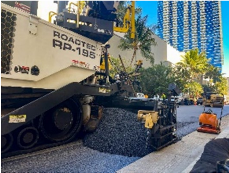
Figure 150. Improper Auger and Tunnel Extensions Cause Segregation
