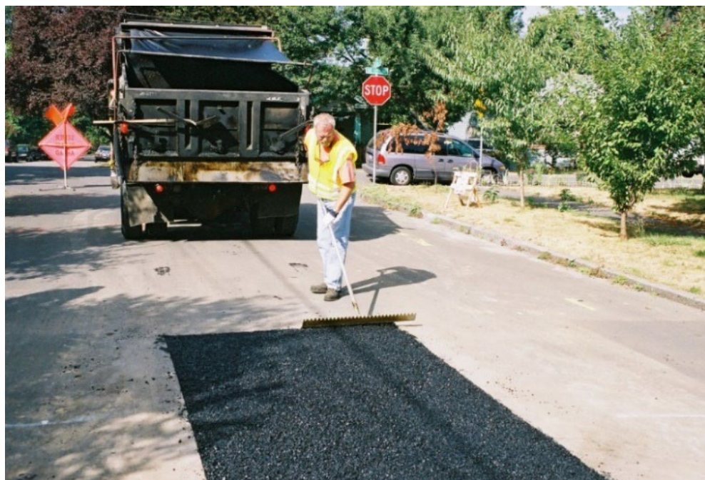
Figure 57. Material Placed in Localized Patch
