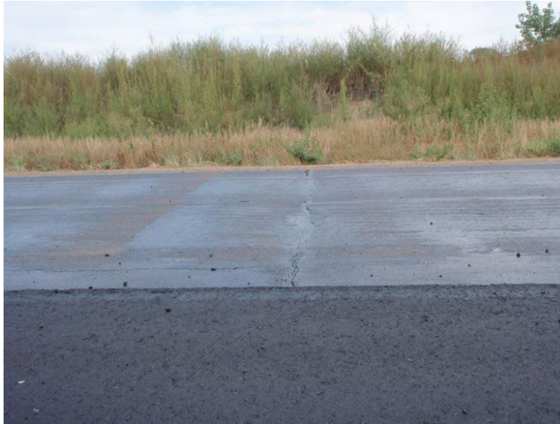
Figure 64. Non-Uniform Application of Tack Coat
