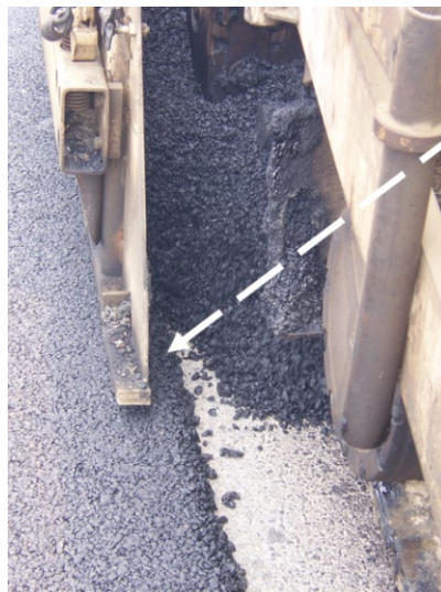
Figure 143. Proper Overlap When Placing the Confined Side of a Longitudinal Joint
