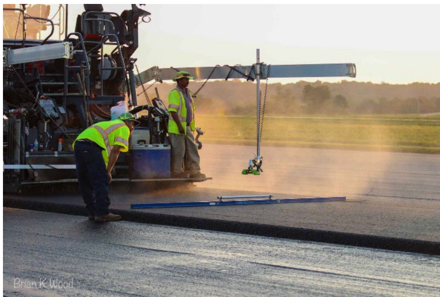
Figure 103. Over-the-Screed Grade Sensor and Cross-Slope Checking
