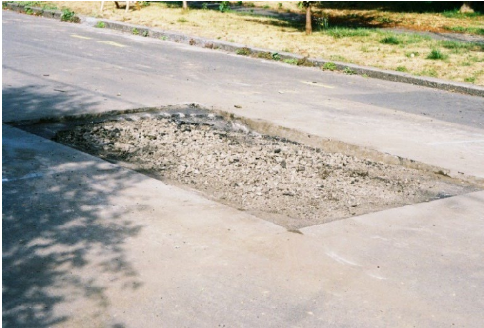
Figure 56. Existing Material Removed Prior to Patching
