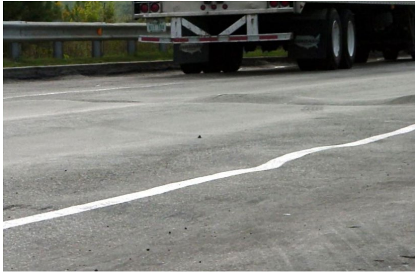
Figure 169. Shoving Due to Unsatisfactory Mix
