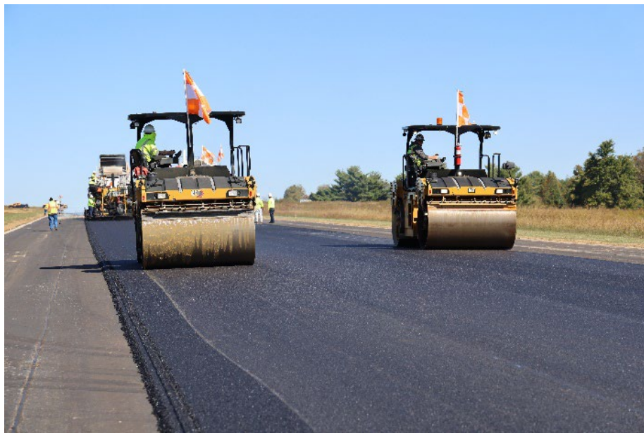
Figure 122. Breakdown Rolling with Multiple Vibratory Rollers
