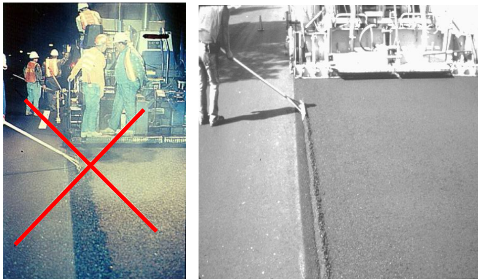
Figure 144. Improper Luting of the LJ (left), which Starves the Hot Side of Rolldown Material, and Proper Luting of the LJ (right)
