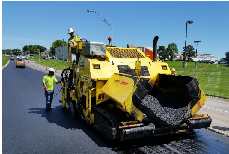
Figure 88. Folding Hopper Wings
