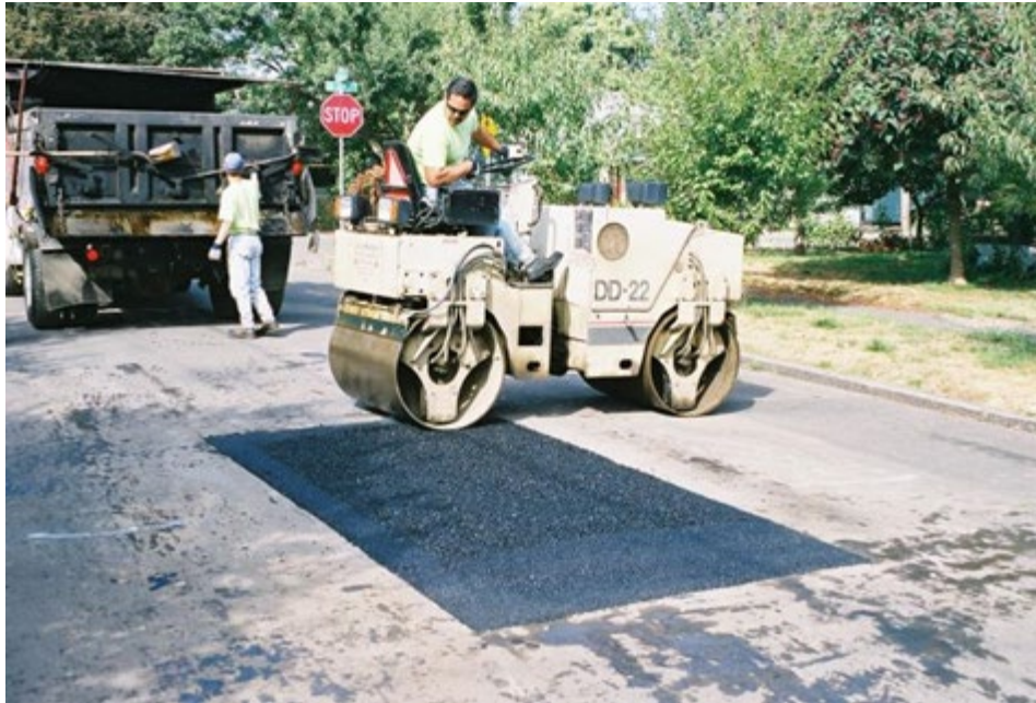
Figure 58. Compaction of Patch
