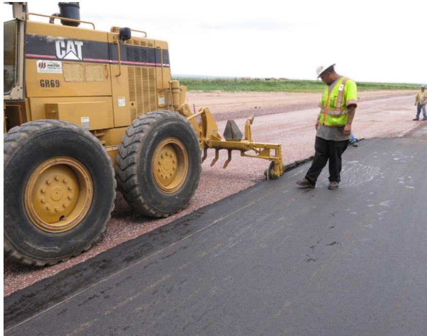
Figure 138. Cutting Wheel Attached to Rear Ripper of a Grader
