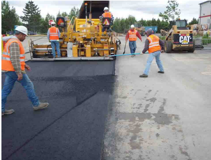
Figure 145. Improper Broadcasting and Luting across the LJ
