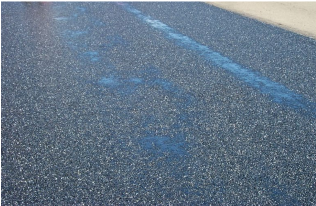
Figure 172. Fat Spot Caused by Localized Excess Asphalt
