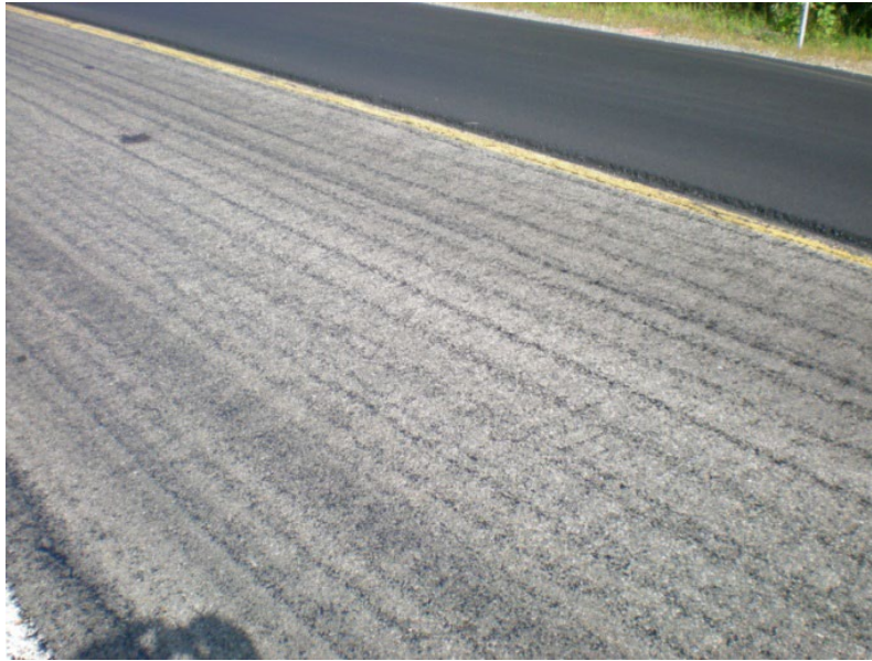
Figure 65. Non-Uniform Application of Tack Coat
