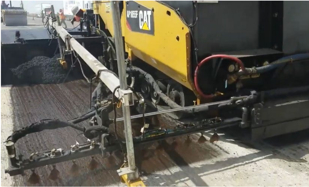
Figure 68. Spray Paver
