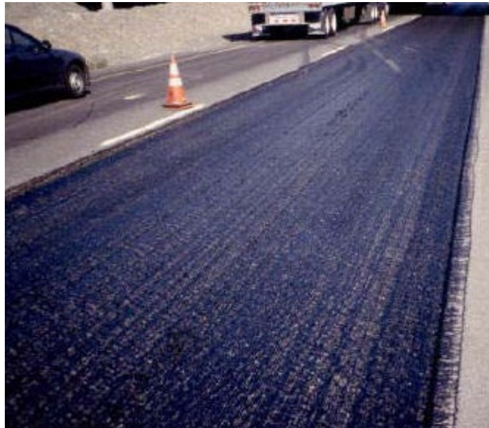
Figure 62. Tack Coat on a Milled Surface
