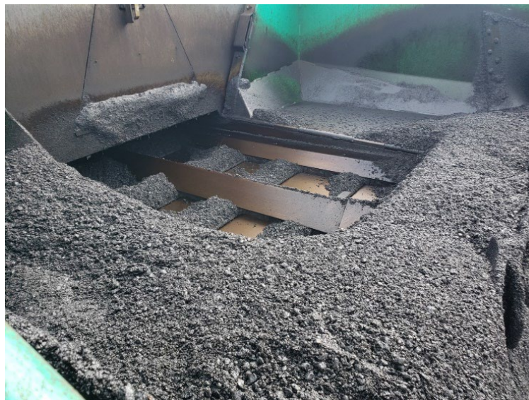
Figure 89. Poorly Managed Paver Hopper
