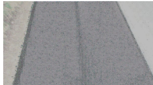
Figure 152. Examples of Centerline Segregation
