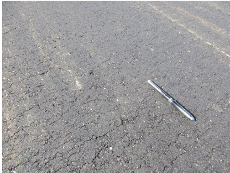
Figure 168. Hairline Cracks Caused by Roller Checking
