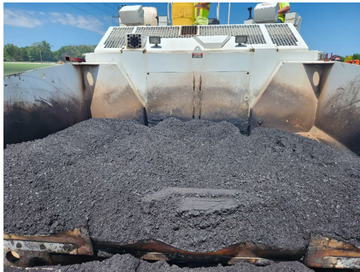
Figure 81. Paver Hopper Between Loads
