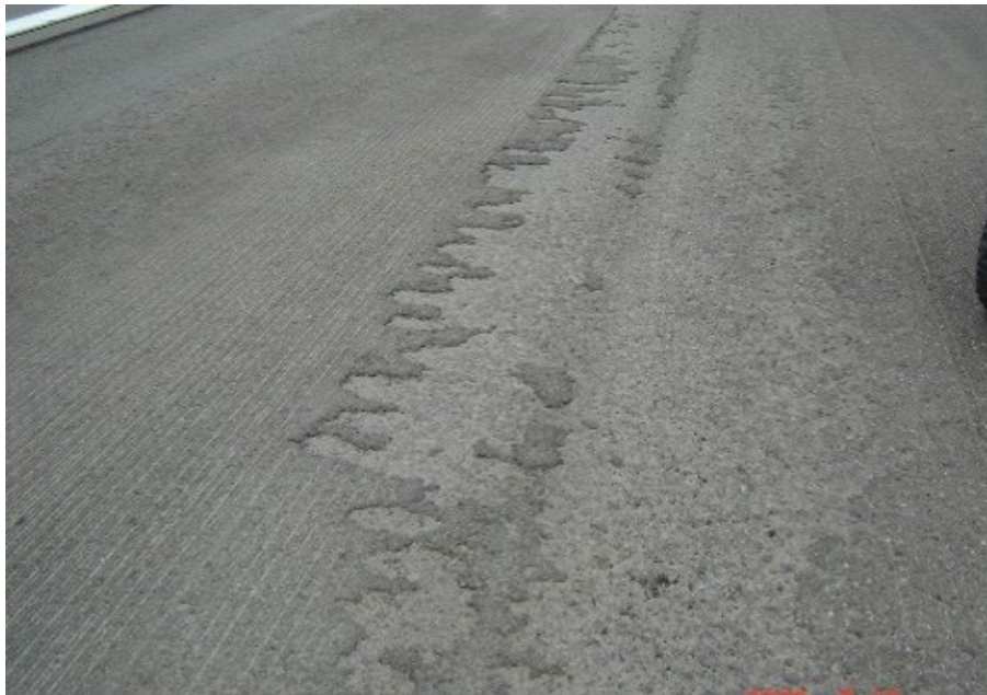
Figure 15. Raveled Asphalt Pavement Surface
