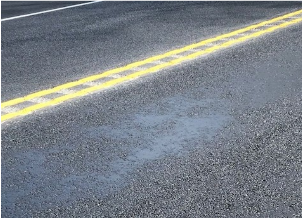
Figure 173. Fat Spot Caused by Fuel Oil Spill Prior to Overlay Construction
