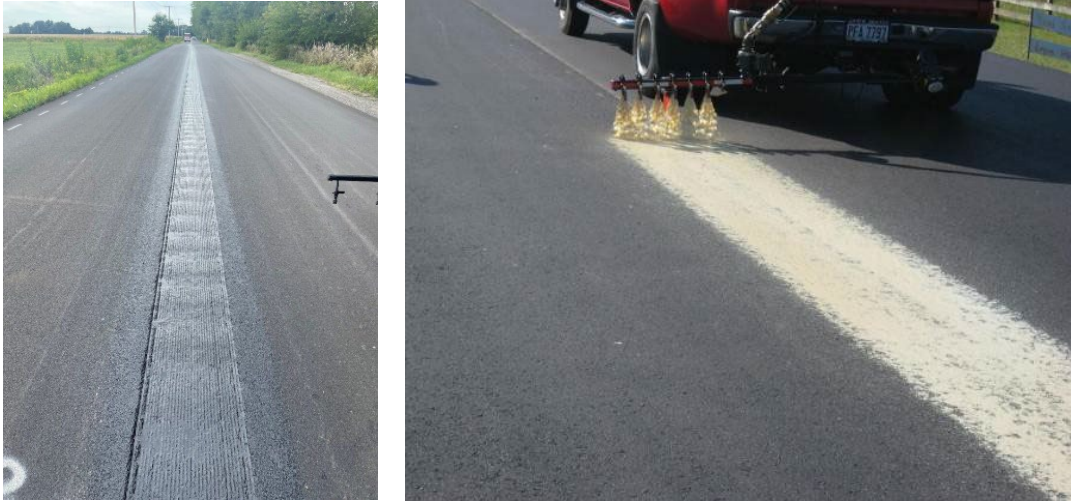
Figure 148. Surface Sealers on LJs: RPE (left) and Rejuvenator VRAM (right)
