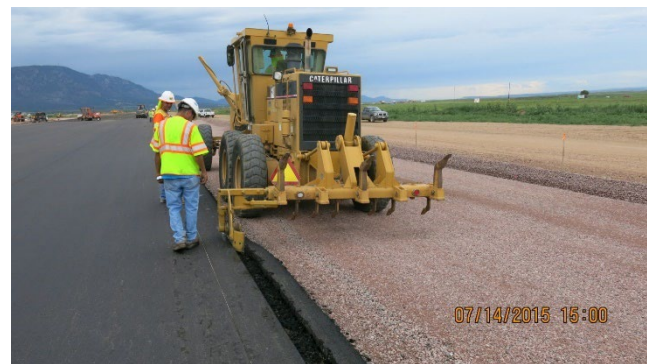
Figure 139. Kick-Out Plate Aids in Removing the Cutback Mix
