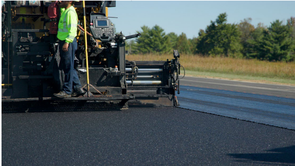
Figure 93. Extendable Screed Paver
