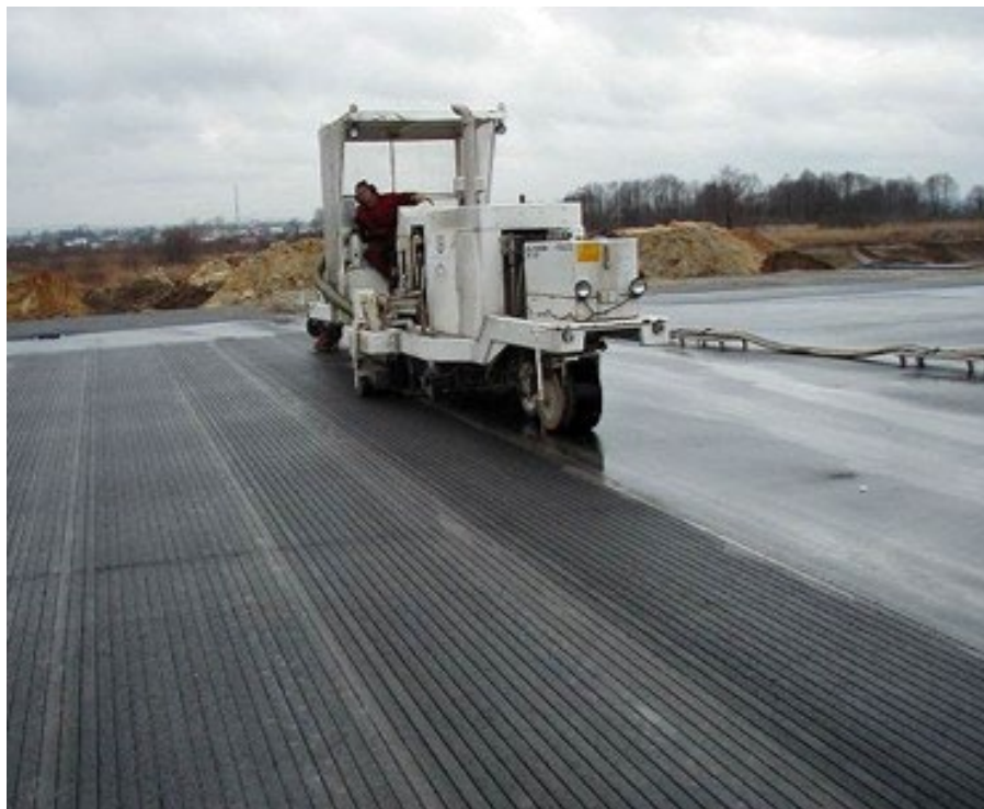
Figure 19. Grooving an Airfield Runway
