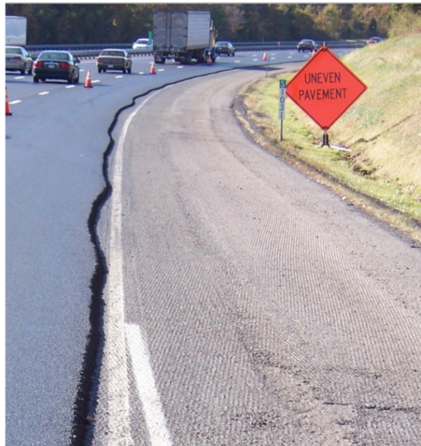
Figure 129. Not Paving Straight (or Smooth on a Curve) Makes It Impossible to Achieve a Consistent Overlay
