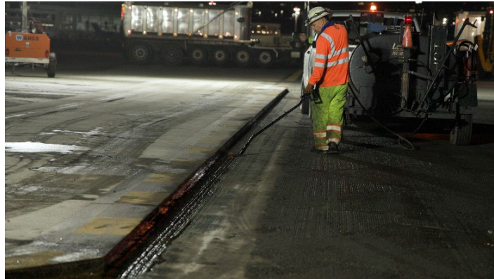
Figure 142. Joint Adhesive Being Applied to the Cold Joint Face
