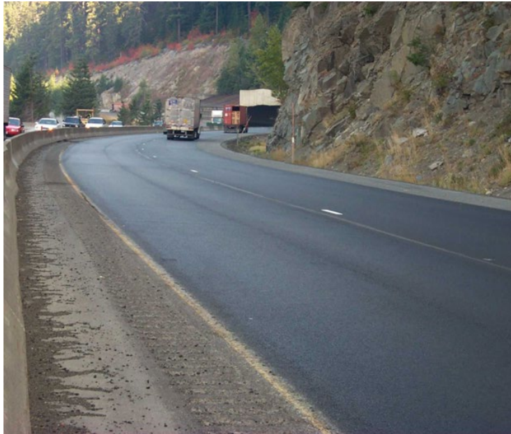
Figure 155. Example of Half-Width Mat Segregation
