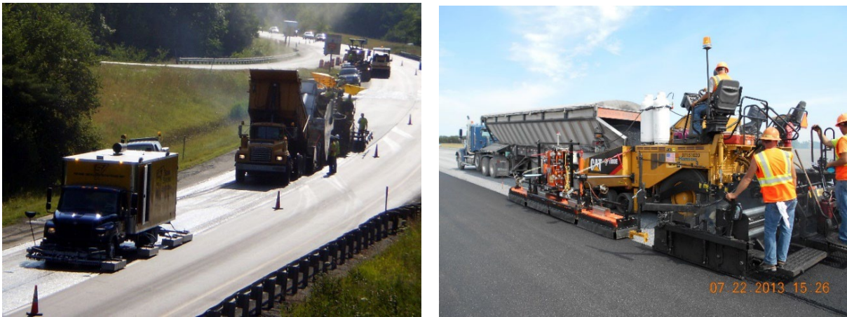
Figure 147. Joint Heaters: Self-Contained (left) and Paver-Mounted (right)
