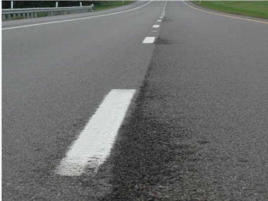
Figure 166. Poor Longitudinal Joint Due to Unsatisfactory Construction
