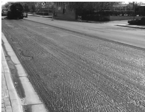
Figure 70. Tack Coat Application
