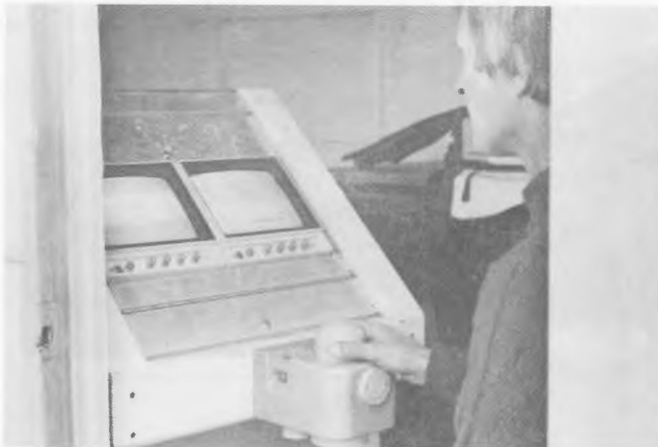
FIGURE 18. OPERATOR AND REMOTE CONTROL DEVICE FOR CINE-SEXTANT MOUNT
