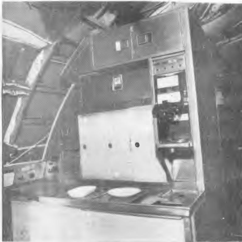
FIGURE 8. AFT GALLEY INSTALLATION
