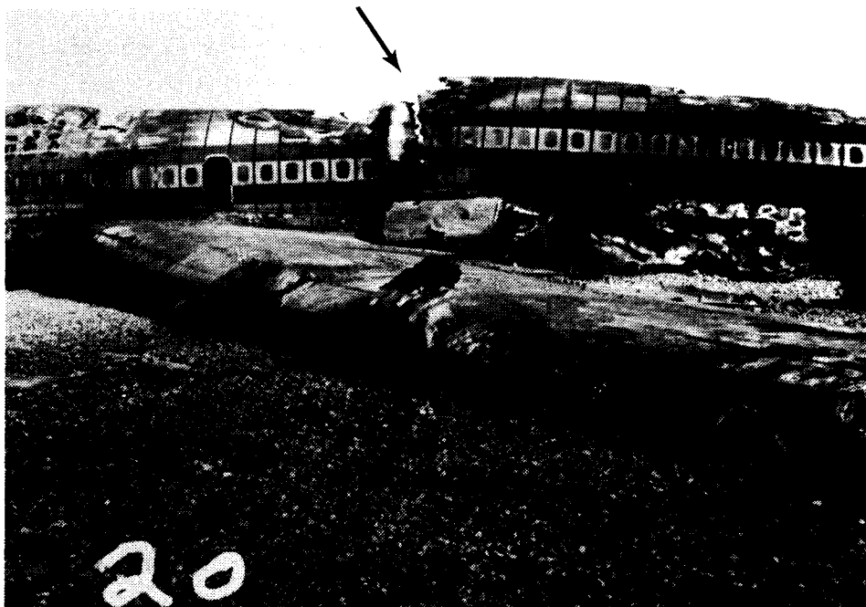
Figure 49. Location of floor break at B.S. 920.
