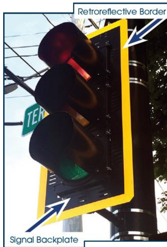
Figure 2.1 Signal Head with a Backplate and Retroreflective Border (FHWA, 2021)
