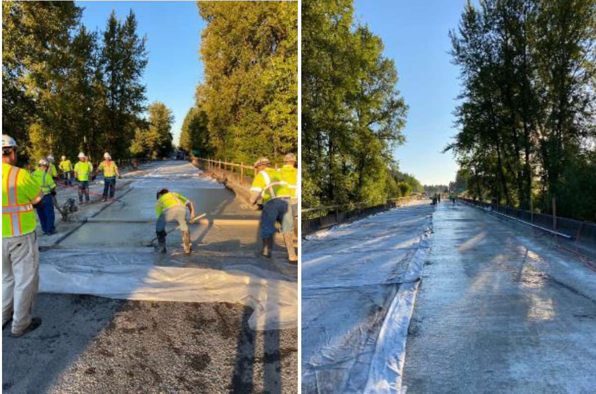
Figure 4-32. Final finishing and curing of Yamhill Crossing bridge deck (BR# 08492), July 26, 2020
