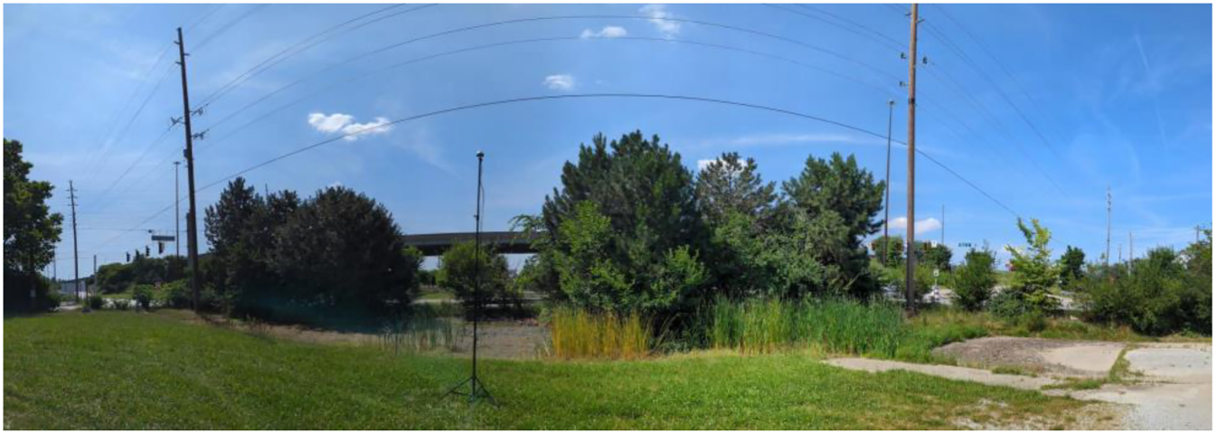
Figure 5.11 RSU Placement for I-70 Ramp Testing.
