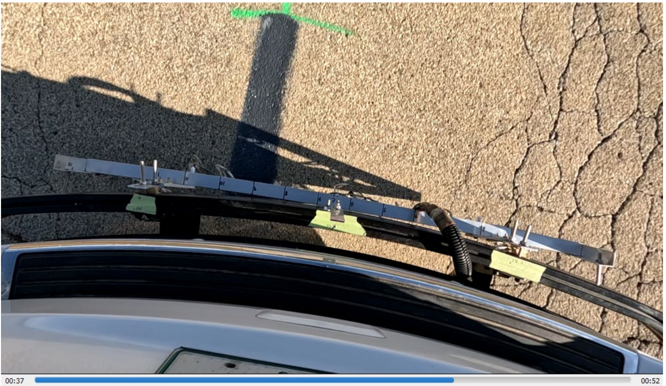
Figure 165. Photo. Referenced photo for longitudinal strip #21 (Case #17).
