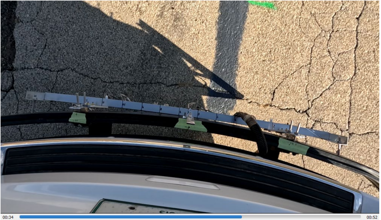
Figure 160. Photo. Referenced photo for longitudinal strip #16 (Case #17).
