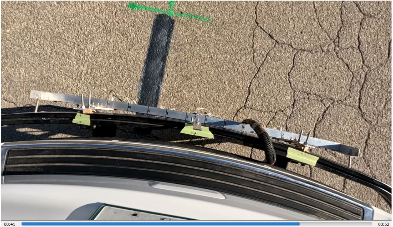
Figure 174. Photo. Referenced photo for longitudinal strip #30 (Case #17).
