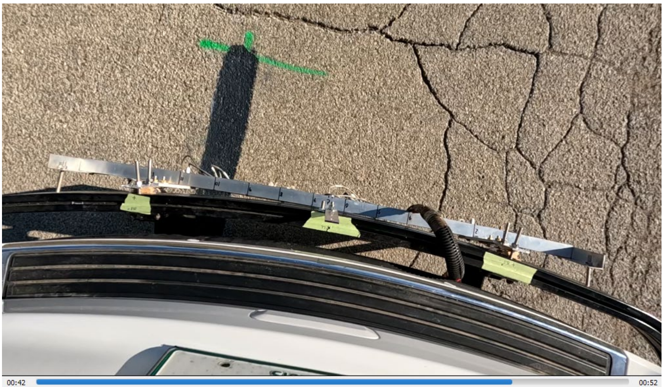
Figure 175. Photo. Referenced photo for longitudinal strip #31 (Case #17).
