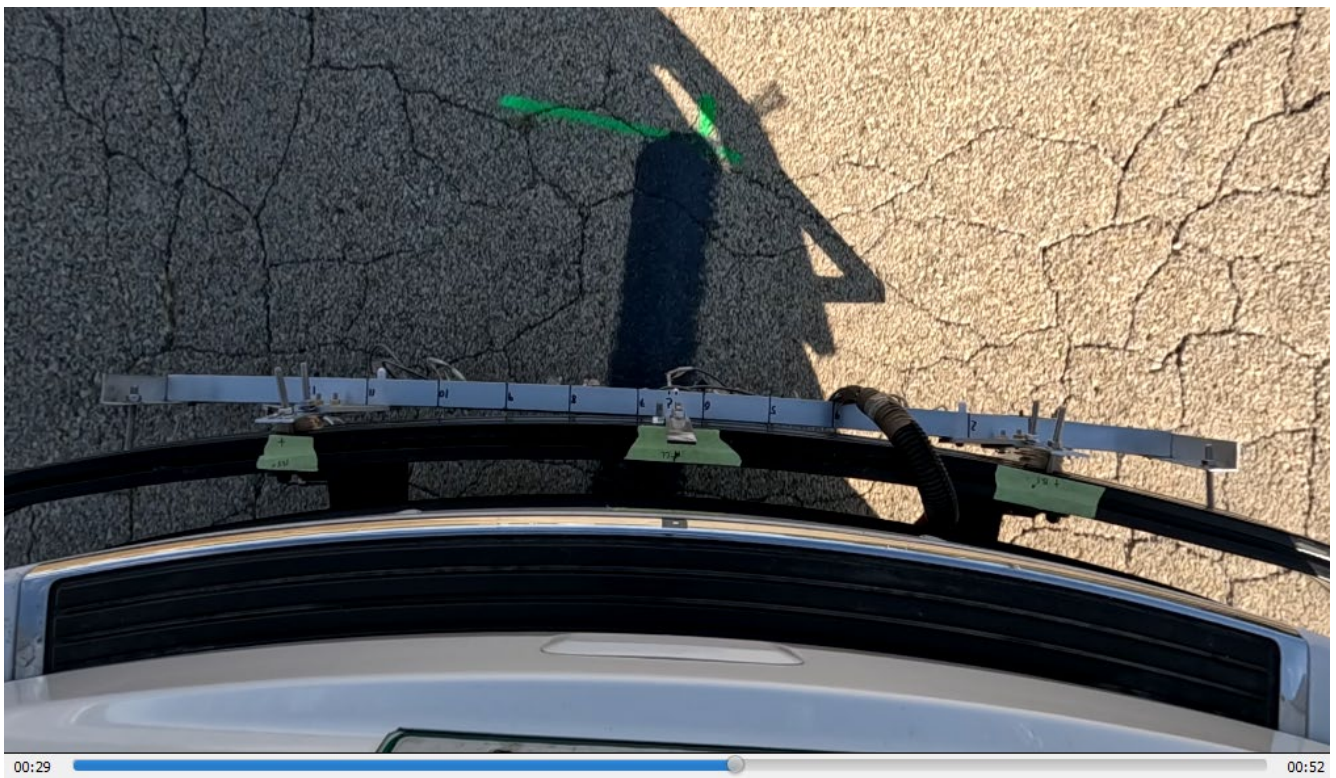
Figure 151. Photo. Referenced photo for longitudinal strip #7 (Case #17).
