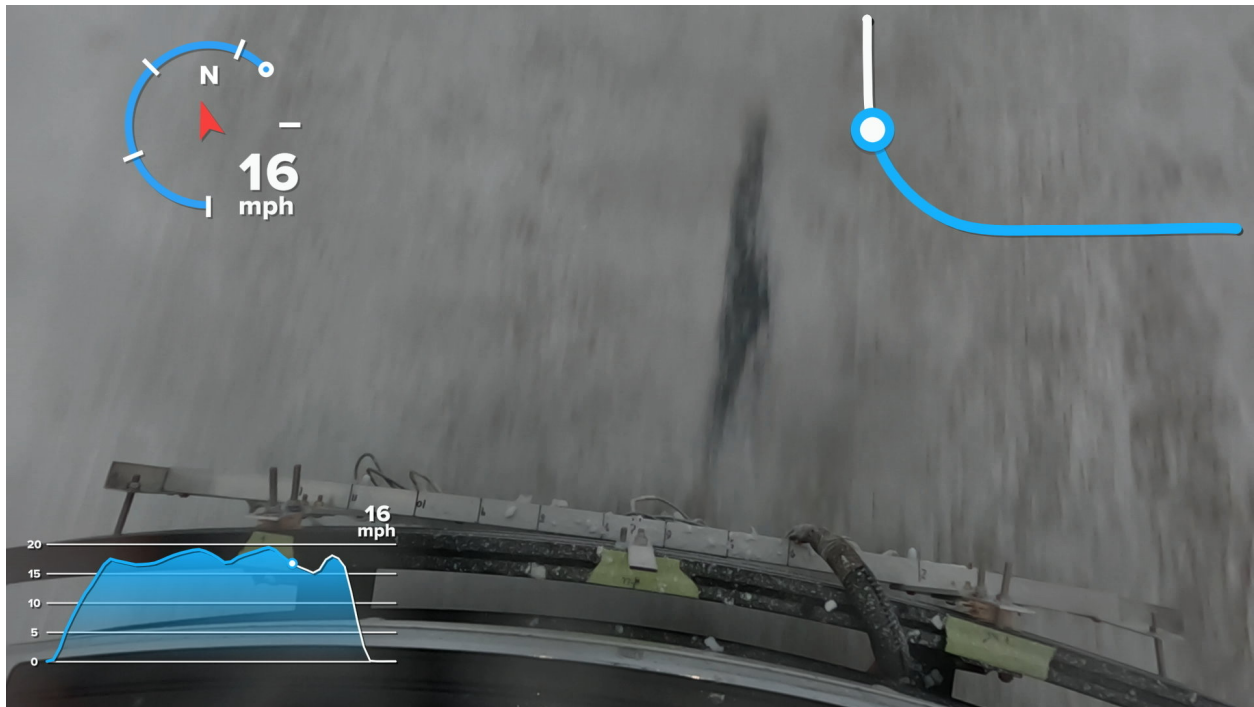
Figure 227. Photo. Referenced photo for longitudinal strip #35 (Case #21).
