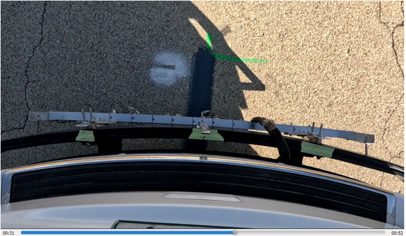
Figure 154. Photo. Referenced photo for longitudinal strip #10 (Case #17).
