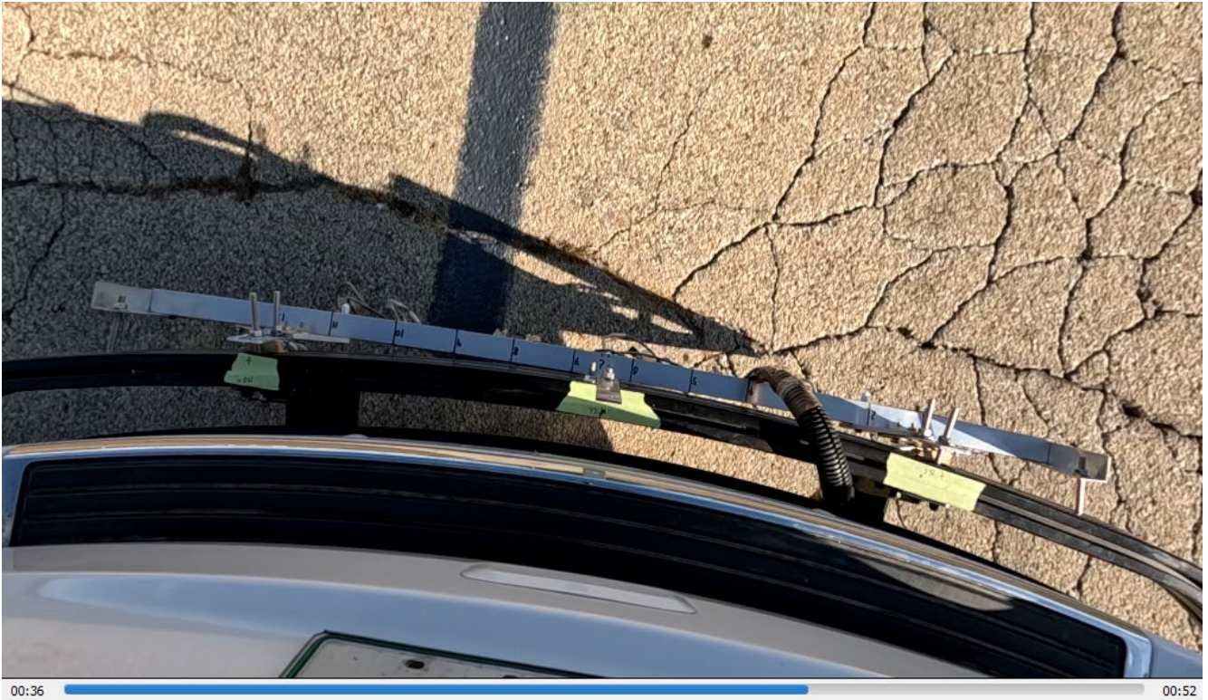
Figure 164. Photo. Referenced photo for longitudinal strip #20 (Case #17).
