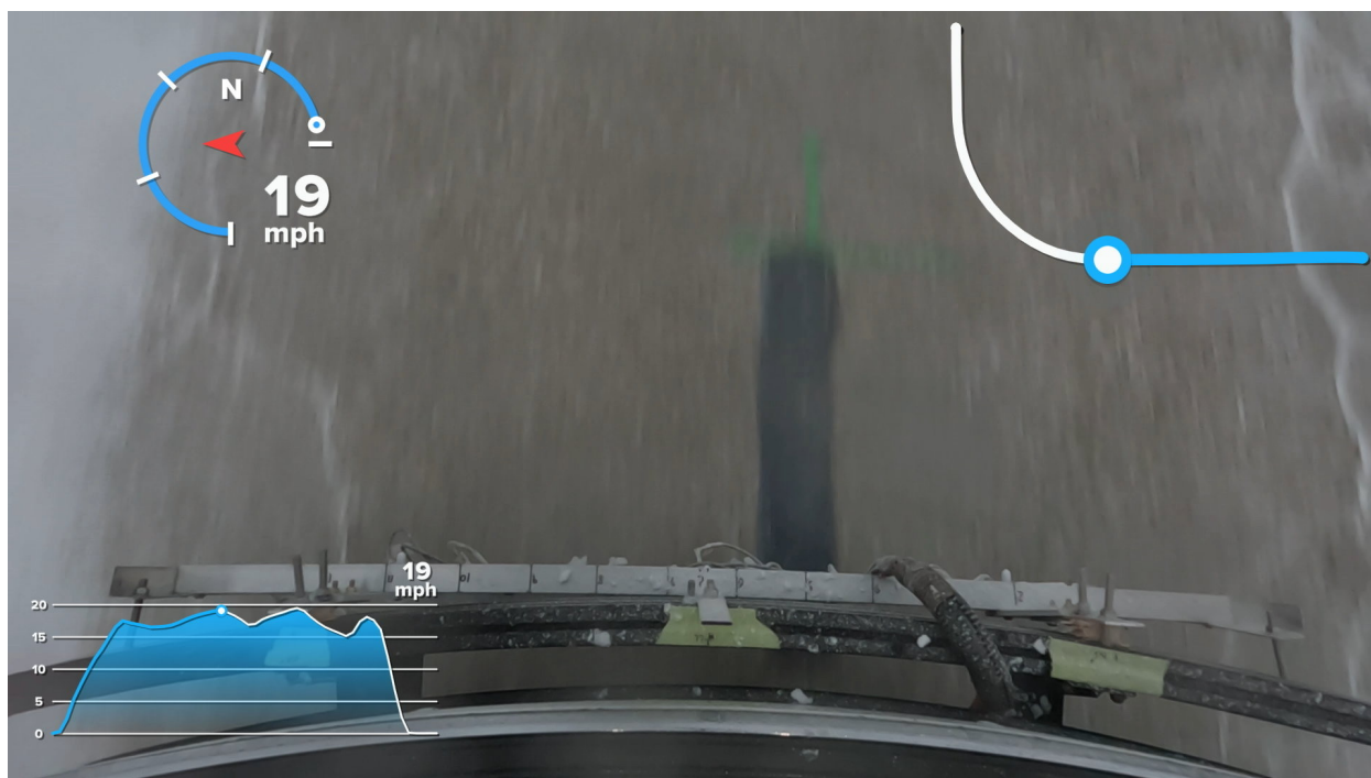
Figure 201. Photo. Referenced photo for longitudinal strip #9 (Case #21).
