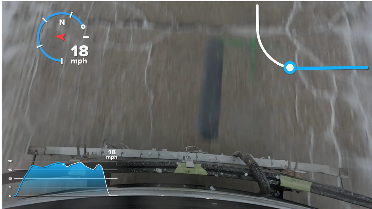
Figure 205. Photo. Referenced photo for longitudinal strip #13 (Case #21).
